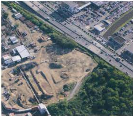
Bechara Industrial Area, Puerto Rico
