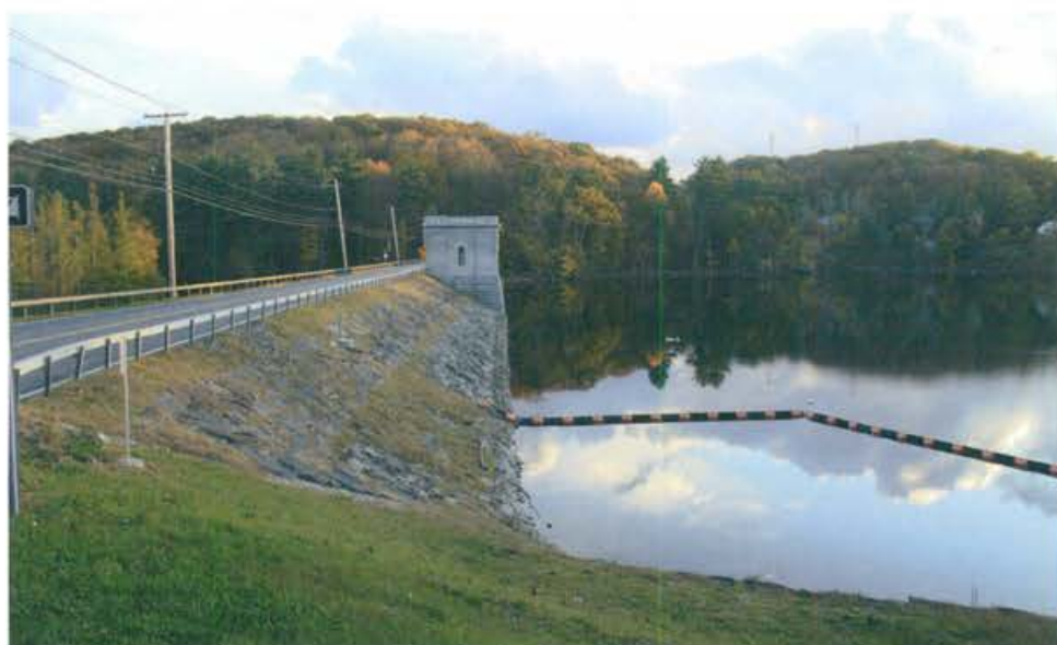
West Branch Dam (1891)
