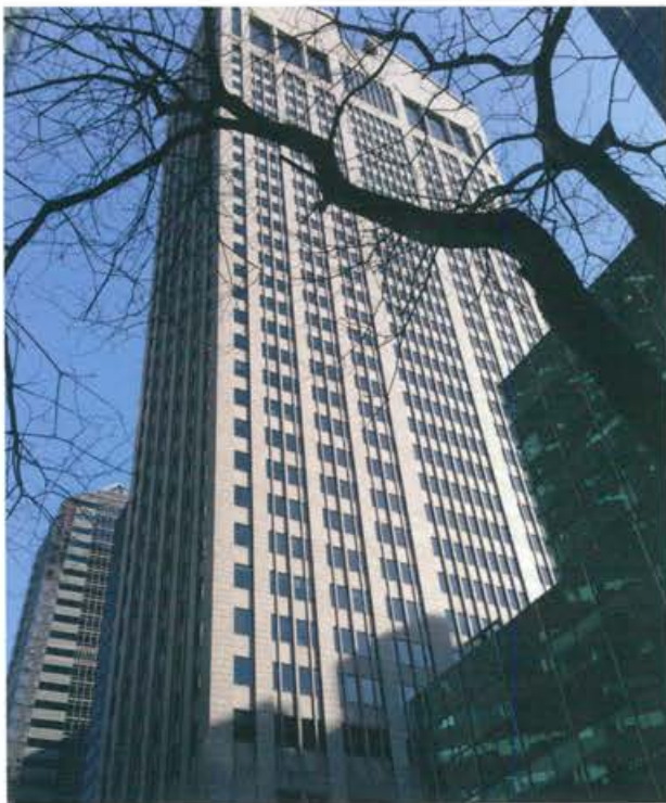
ATT Building (Philip Johnson &amp; John Burgee, 1984)
