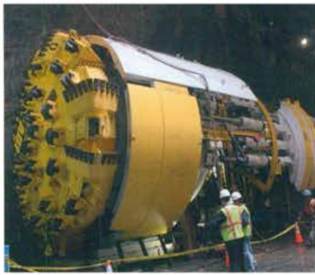
Second Avenue Subway
