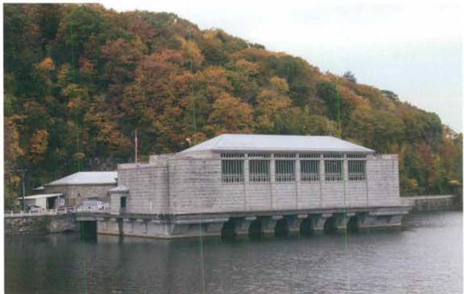
Ultraviolet Disinfection Facility
