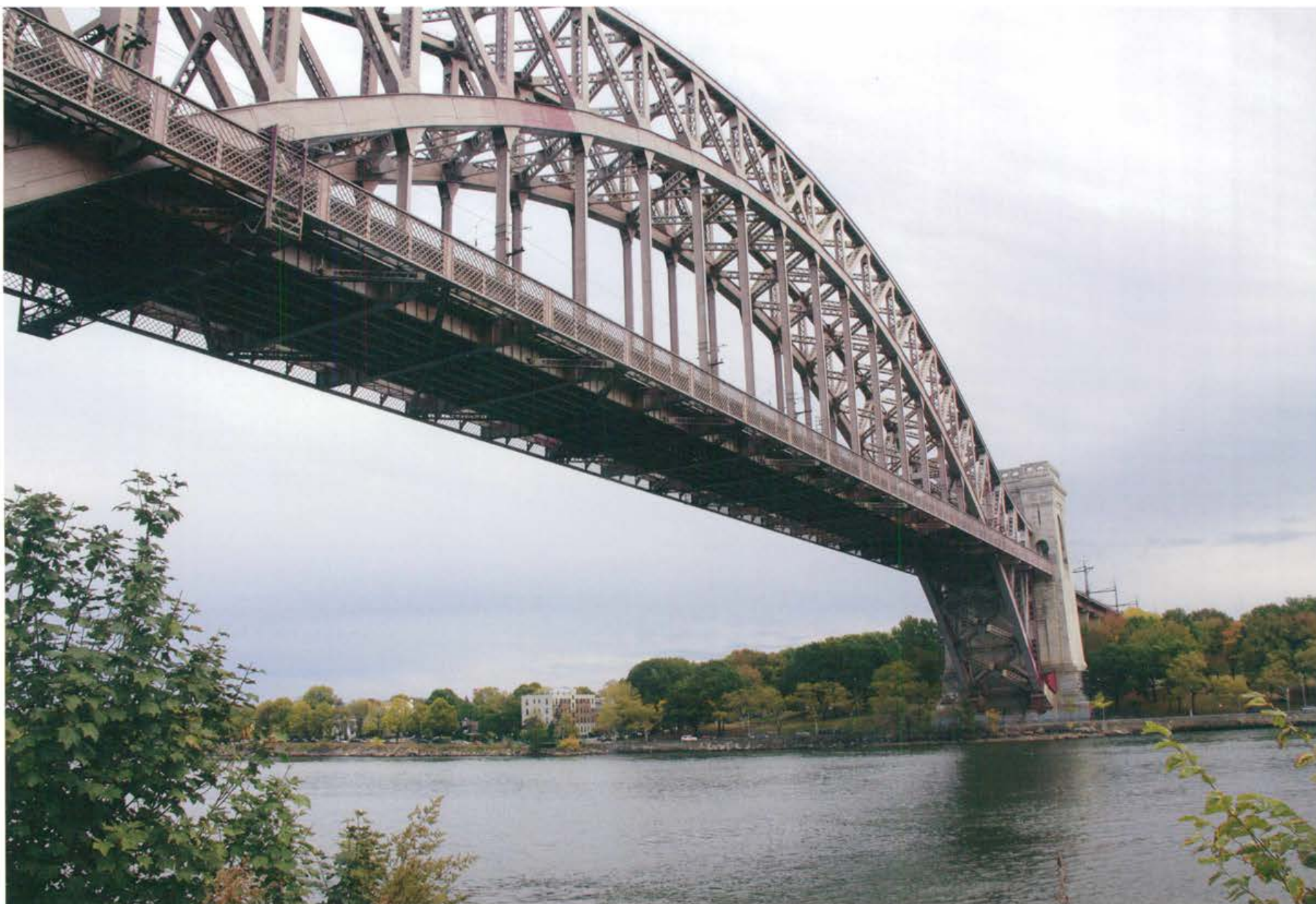
Hell Gate Bridge (Gustav Lindenthal, 1916)
