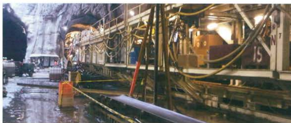
Second Avenue Subway
