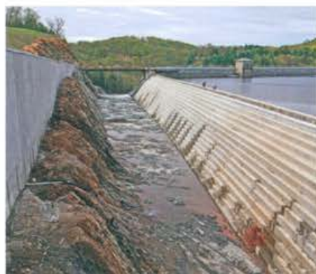
Croton Falls Dam, Westchester County, NY. 2012
