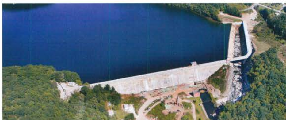
Croton Falls Dam, Westchester County, Nueva York . 2012
