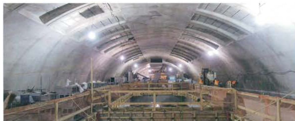
Second Avenue Subway
