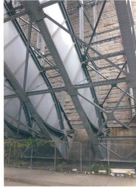
Washington Bridge (Schneider, 1889)
