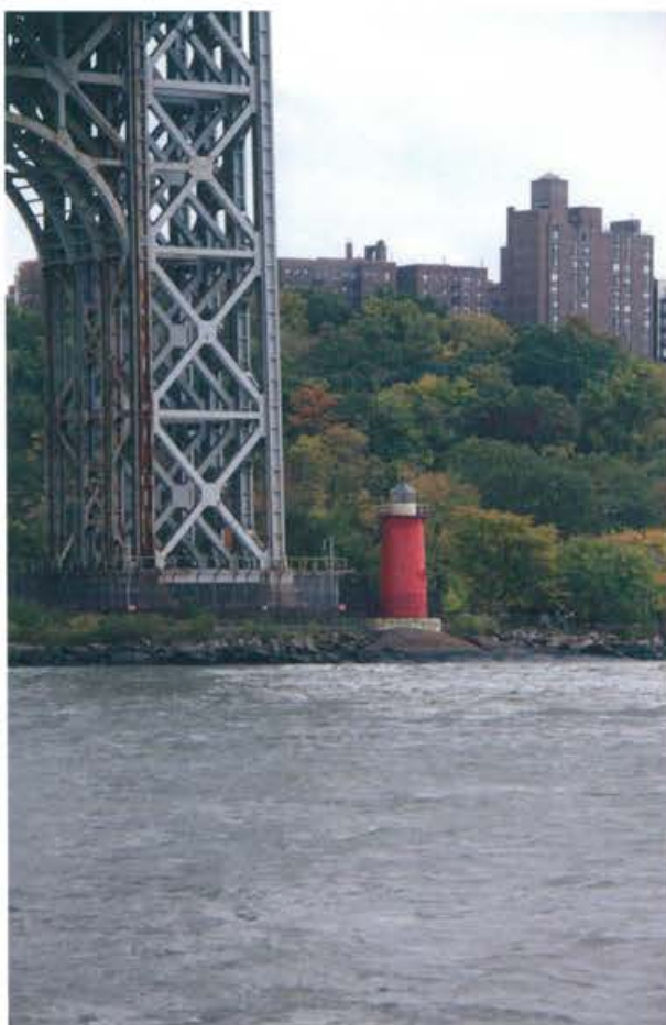
George Washington Bridge
