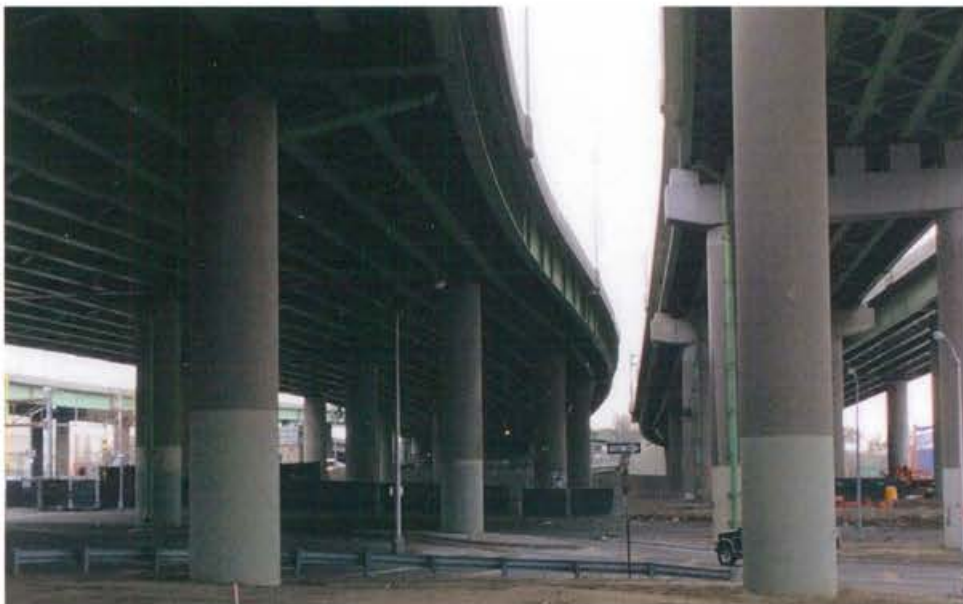
Washington bridge RiversideDR
