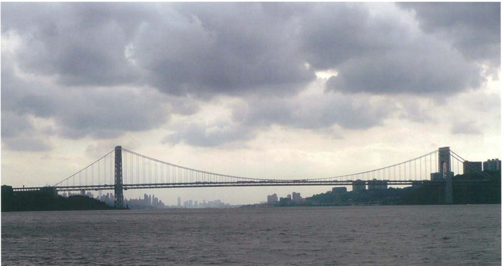
George Washington Bridge
