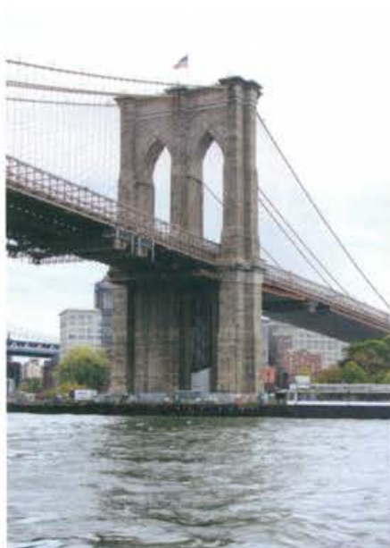
Brooklyn Bridge (Roebling, 1883)
