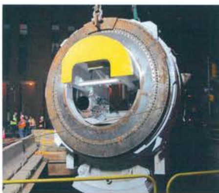
Second Avenue Subway
