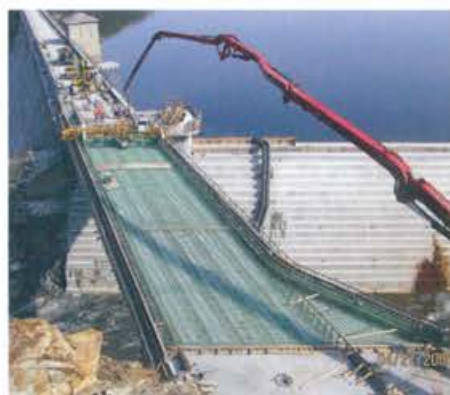
Croton Falls Dam, Westchester County, NY. 2012
