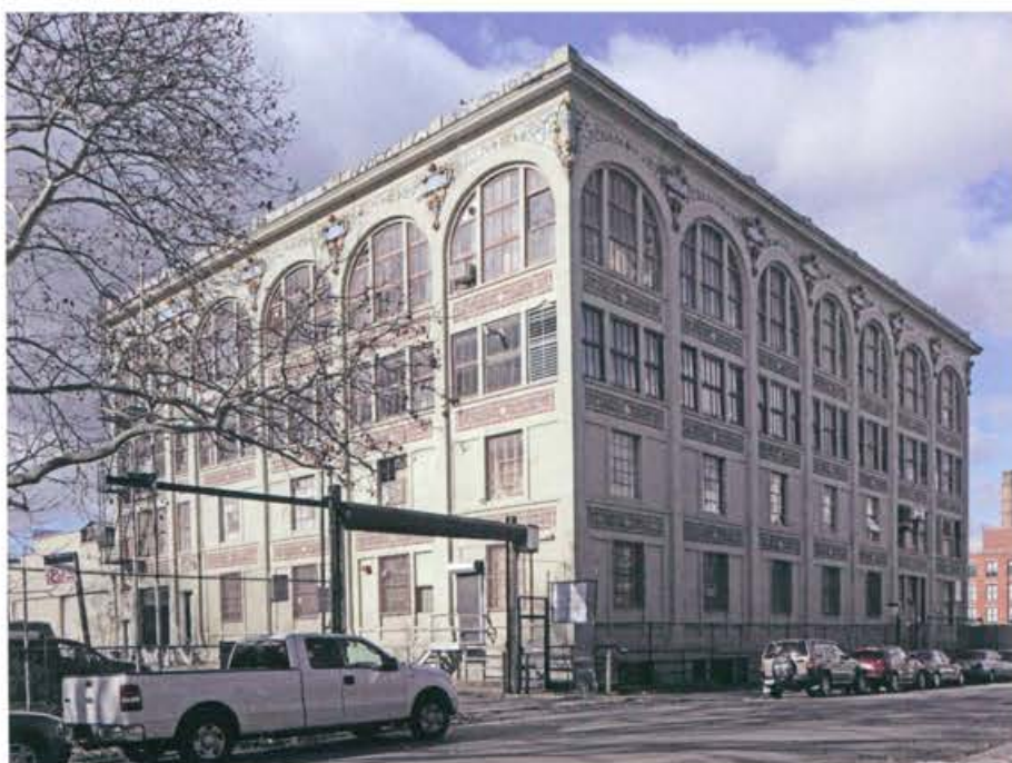
Thomson Meter Company Building (Louis E. Jallade, F. Hennebique, 1908)
