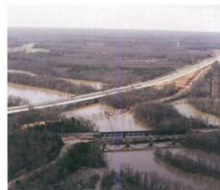
Yadkin River Bridge 2013
