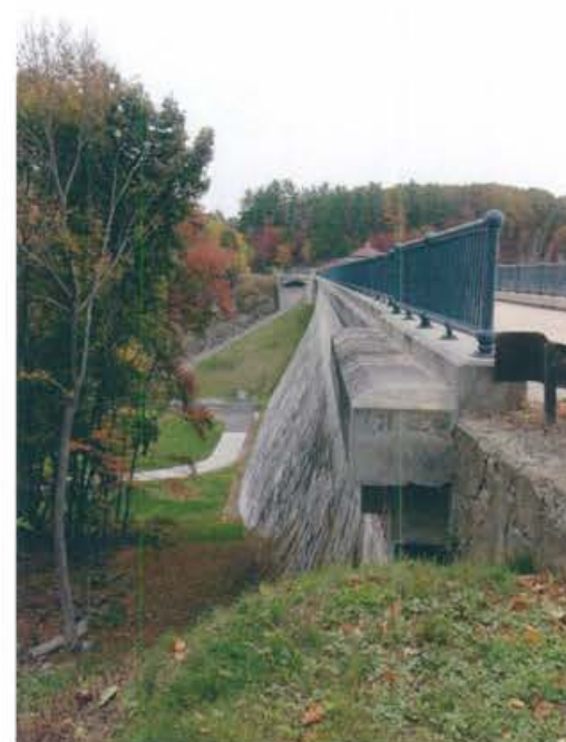
West Branch Dam (1891)
