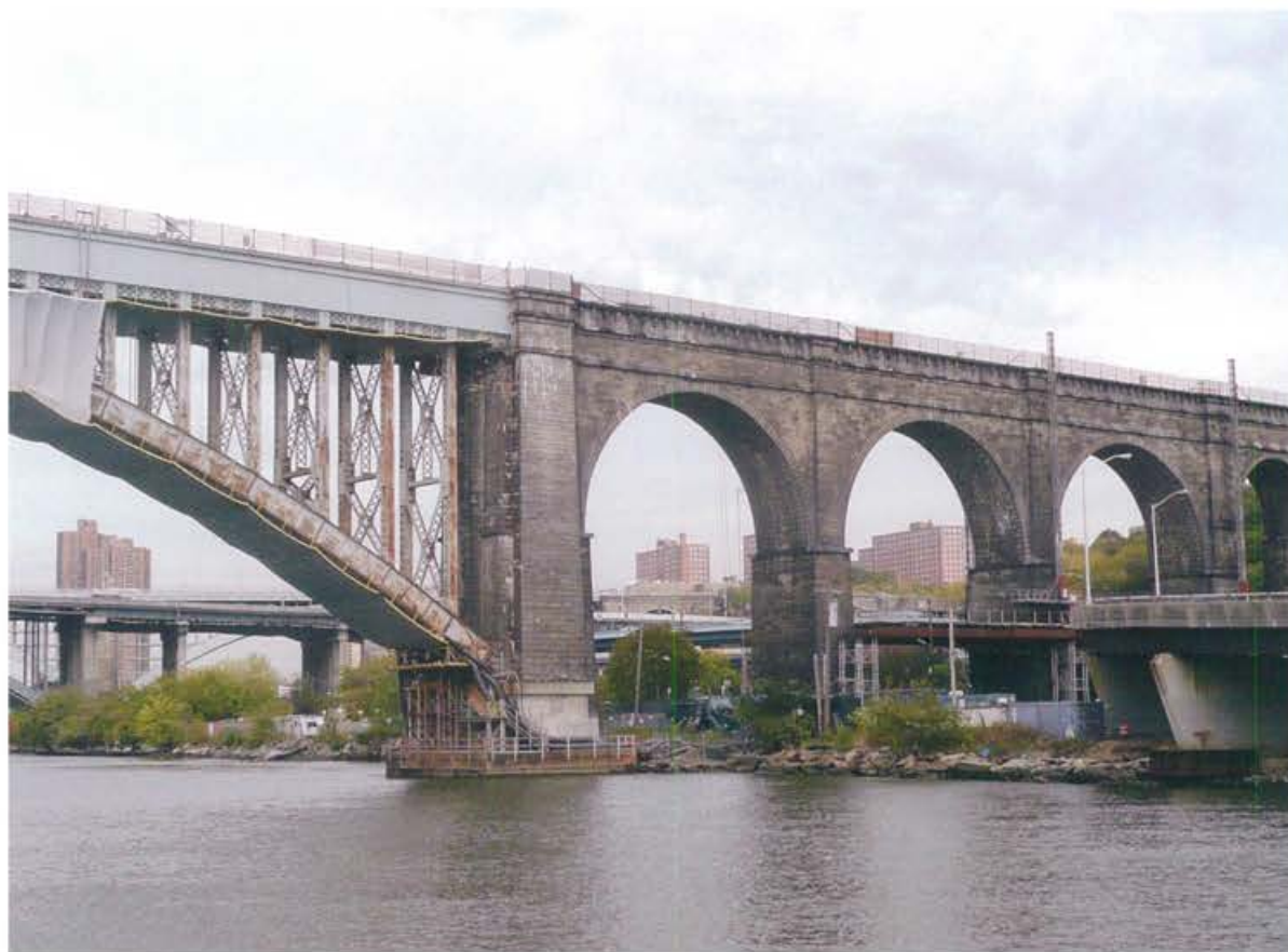
High Bridge Aqueduct (1848) and Tower (1848)
