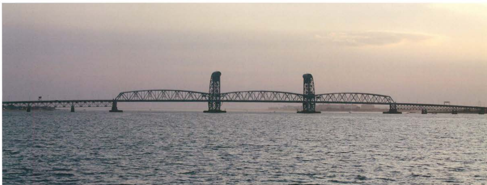
Marine Parkway Bridge
