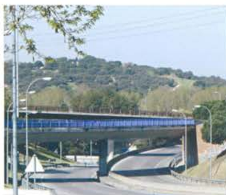
Management of road infrastructures. Link A6 M30, Madrid. 2015
