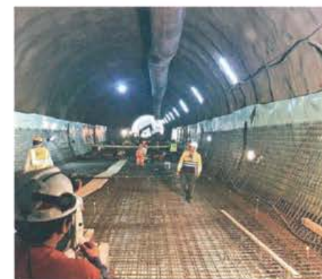
Lima Subway Line 1 Peru. 2016
