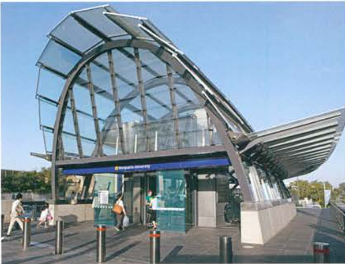
Epping to Chatswood Rail Line 14. Built by ACS, 2009
