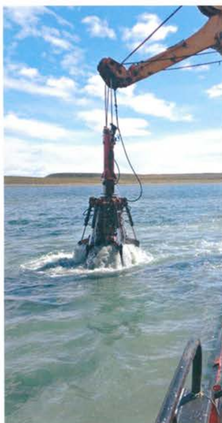
Dredging of Chilota Bay, Chile. 2014
