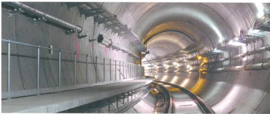
Epping to Chatswood Rail Line
