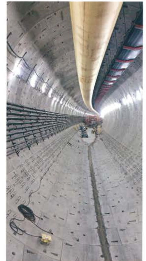
Seattle Tunnel, USA. 2016
