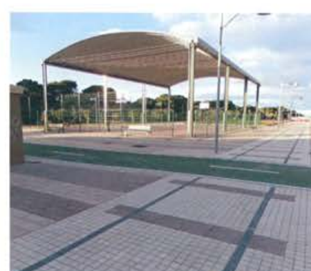
Pinar de Antequera housing complex, Valladolid. 2015
