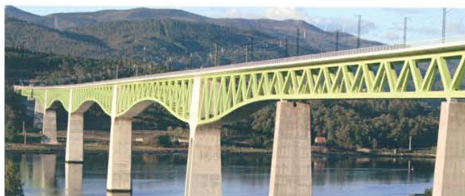
Viaduct over the Ulla river, Pontevedra. 2015
