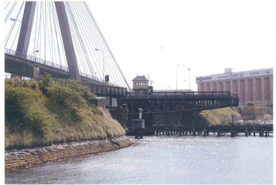
Open section of the old Glebe Swing Bridge
