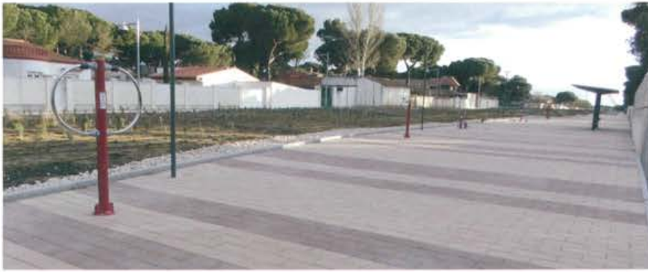
Pinar de Antequera housing complex, Valladolid. 2015
