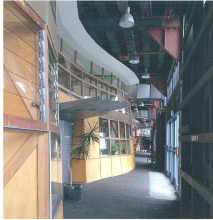
Rehabilitation of Walsh Bay Fingers, Access points and Theater
