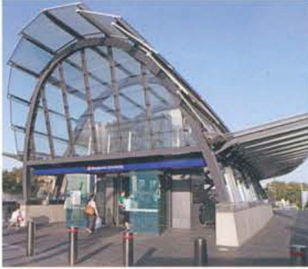
Epping to Chatswood Rail Line 14
