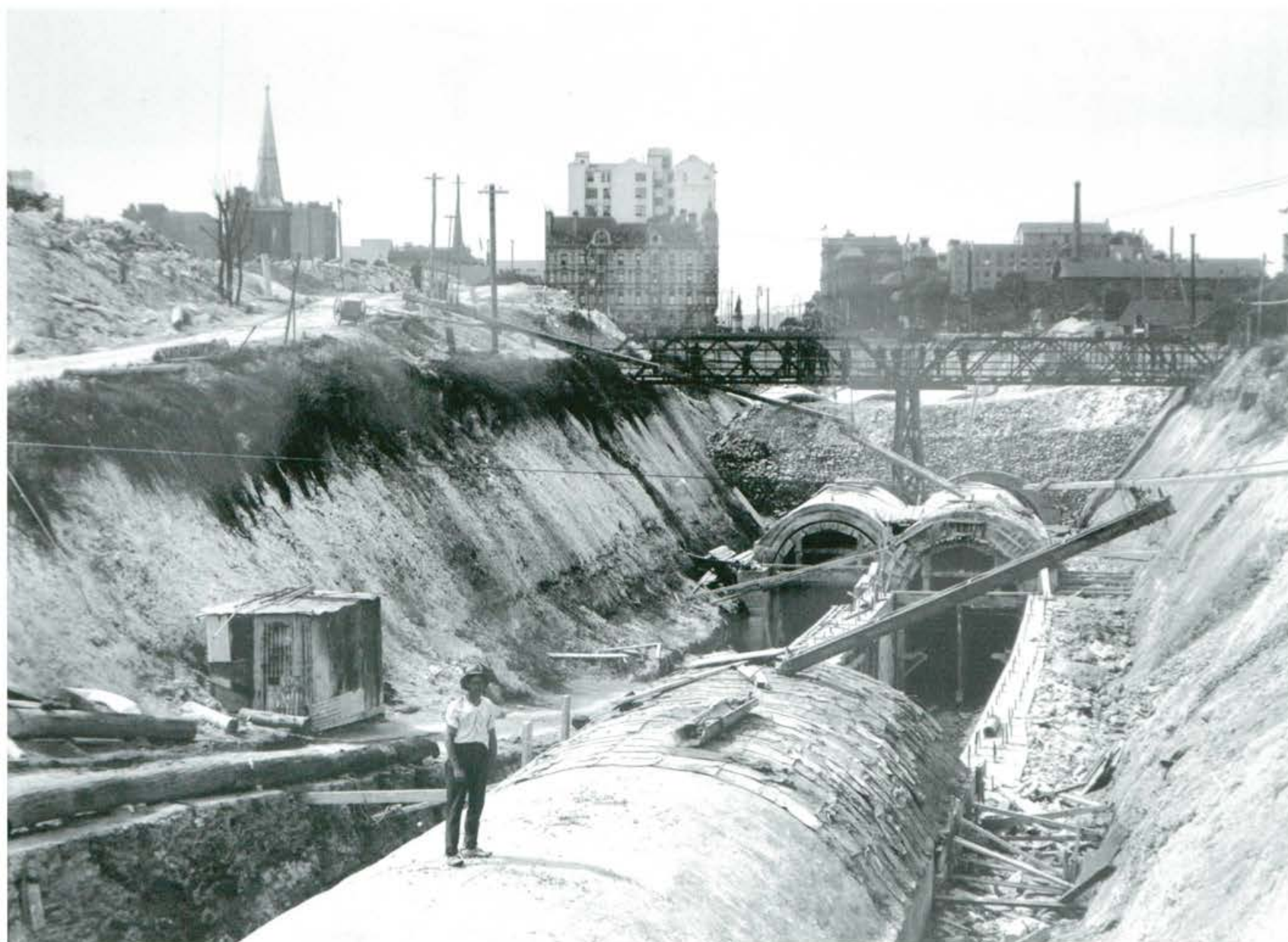
City Railway construction, tunnels leading to St James station, taken in 1924. Courtesy of Australian Railway Historical Society, Railway Resource Centre, 507097
