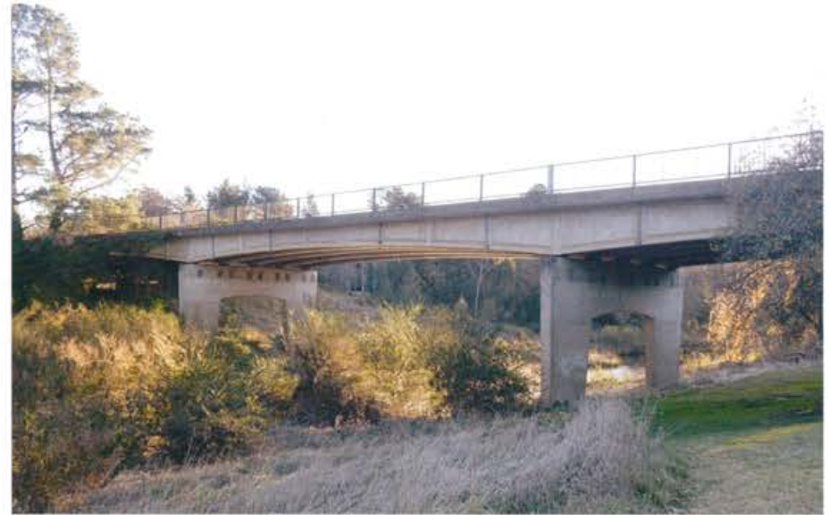
Berrima Bridge over Wingecarribee River
