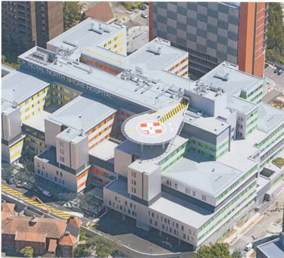
Royal North Shore Hospital Infrashore
