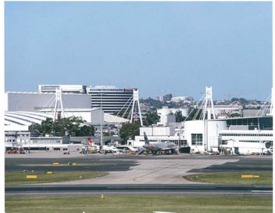
Sydney International Airport
