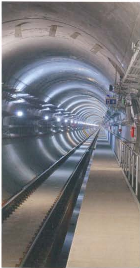
Epping to Chatswood Rail Line
