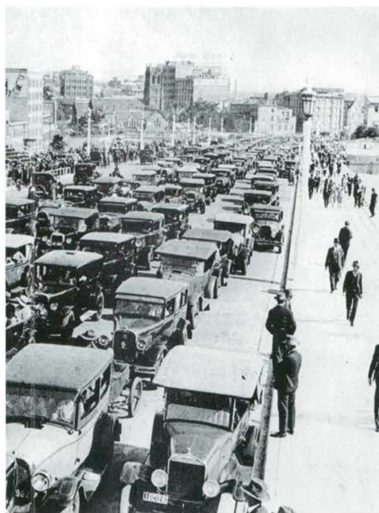
One million delighted people cross the bridge on its inauguration day [59:23]
