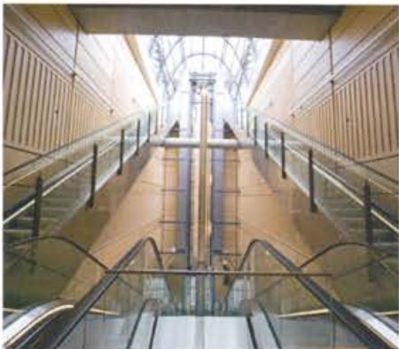
Epping to Chatswood Rail Line
