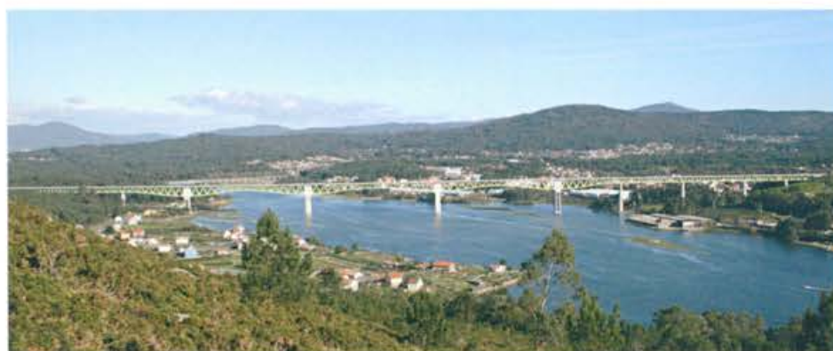
Viaduct over the Ulla river, Pontevedra. 2015
