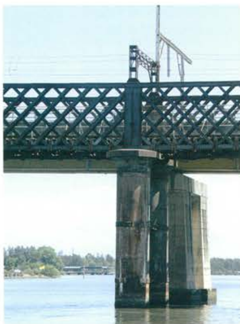
John Whitton Bridge in Rhodes over Parramatta River
