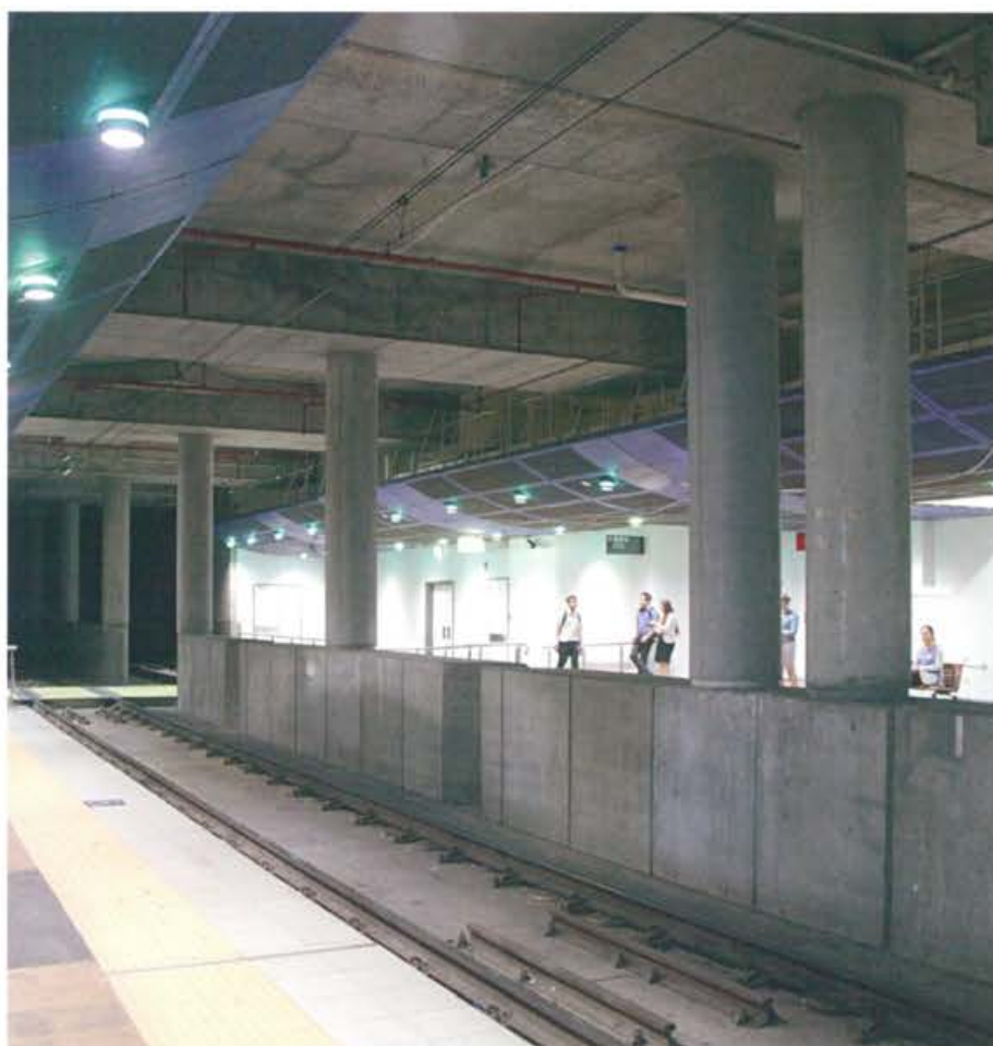
Light Rail en Central Station (1997)
