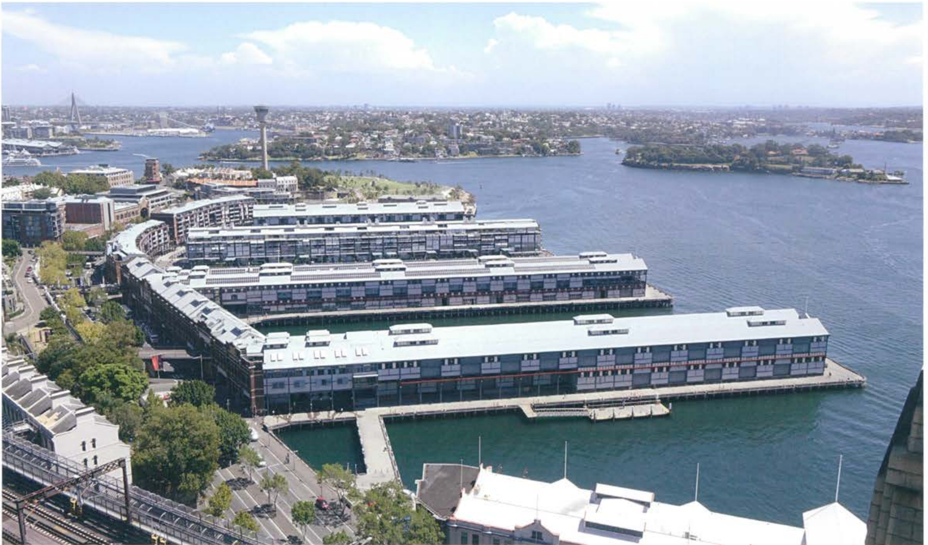
Rehabilitation of Walsh Bay Fingers
