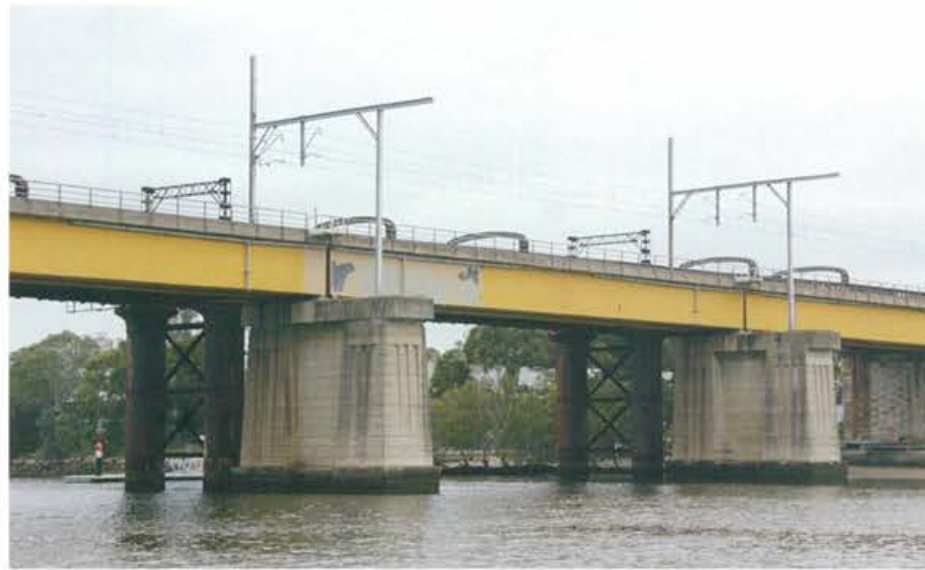
Meadowbank Rail Bridge, 1885
