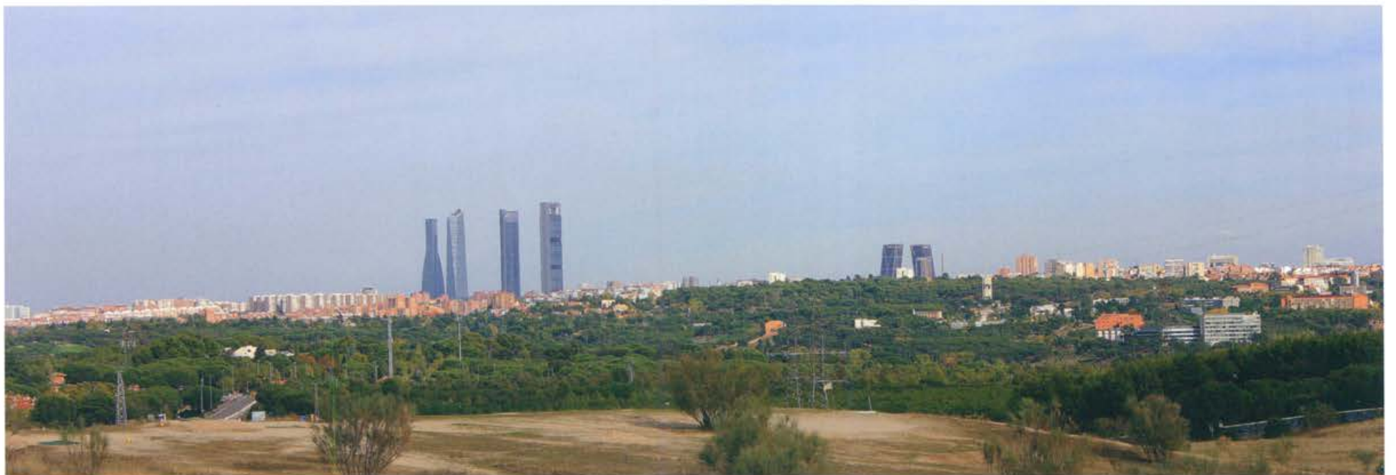
Current skyline of Madrid from the Casa de Campo: the Castellana towers
