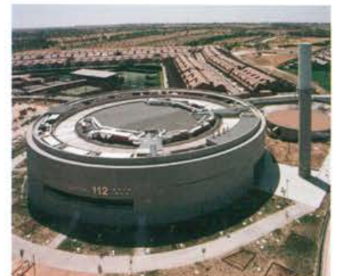
Community of Madrid Emergency Centre
