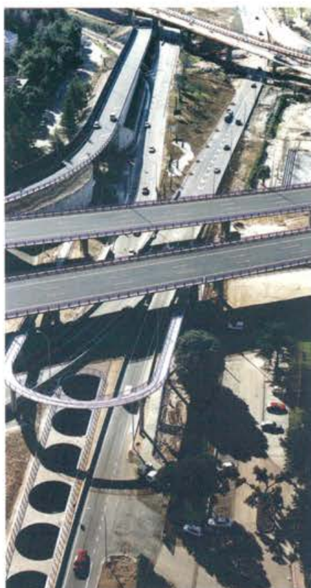
El Pardo junction footbridge, M-30 and M-40
