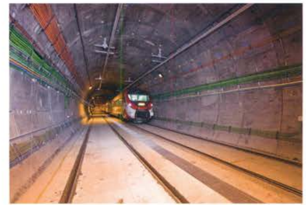
Puerta del Sol, new Suburban rail station
