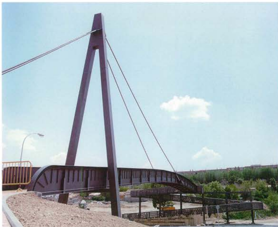
Footbridge on the Calle Sinesio Delgado, Madrid (Jiménez Cañas, 2008)
