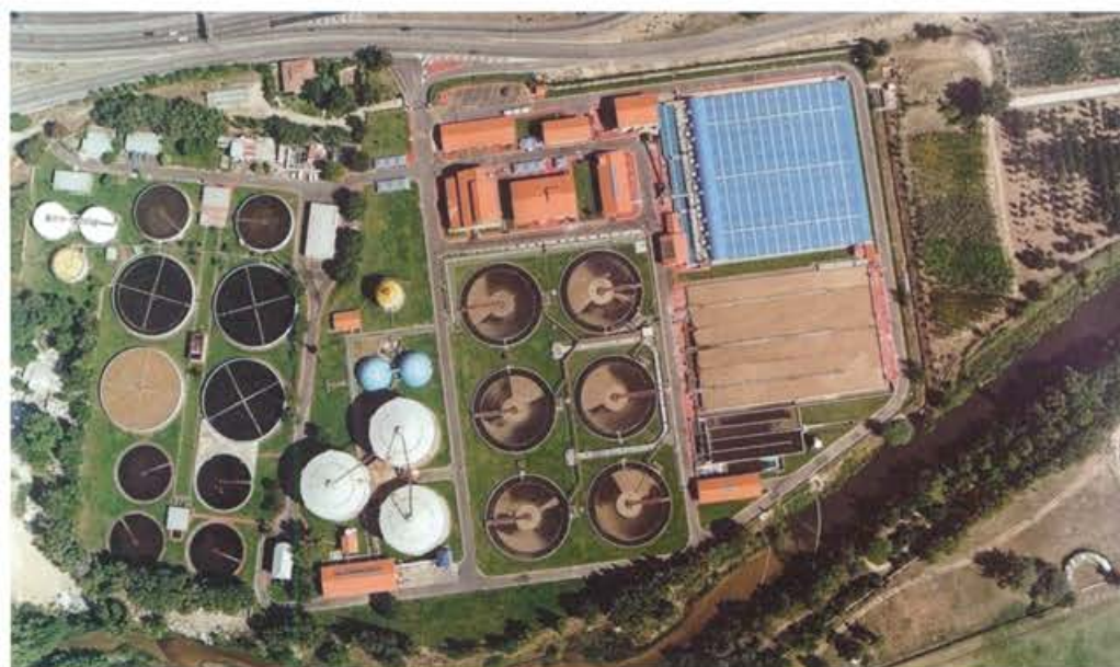
Viveros (Madrid) waste water treatment plant
