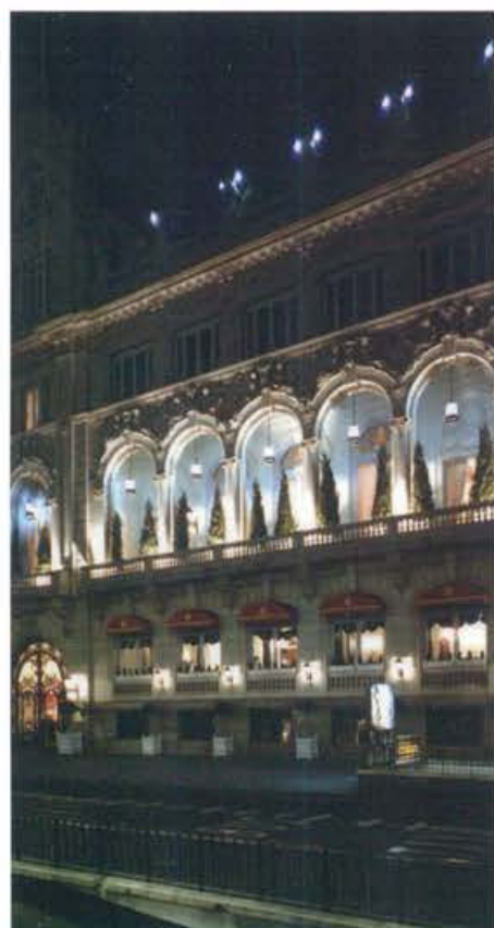
Madrid Casino [Restoration]
