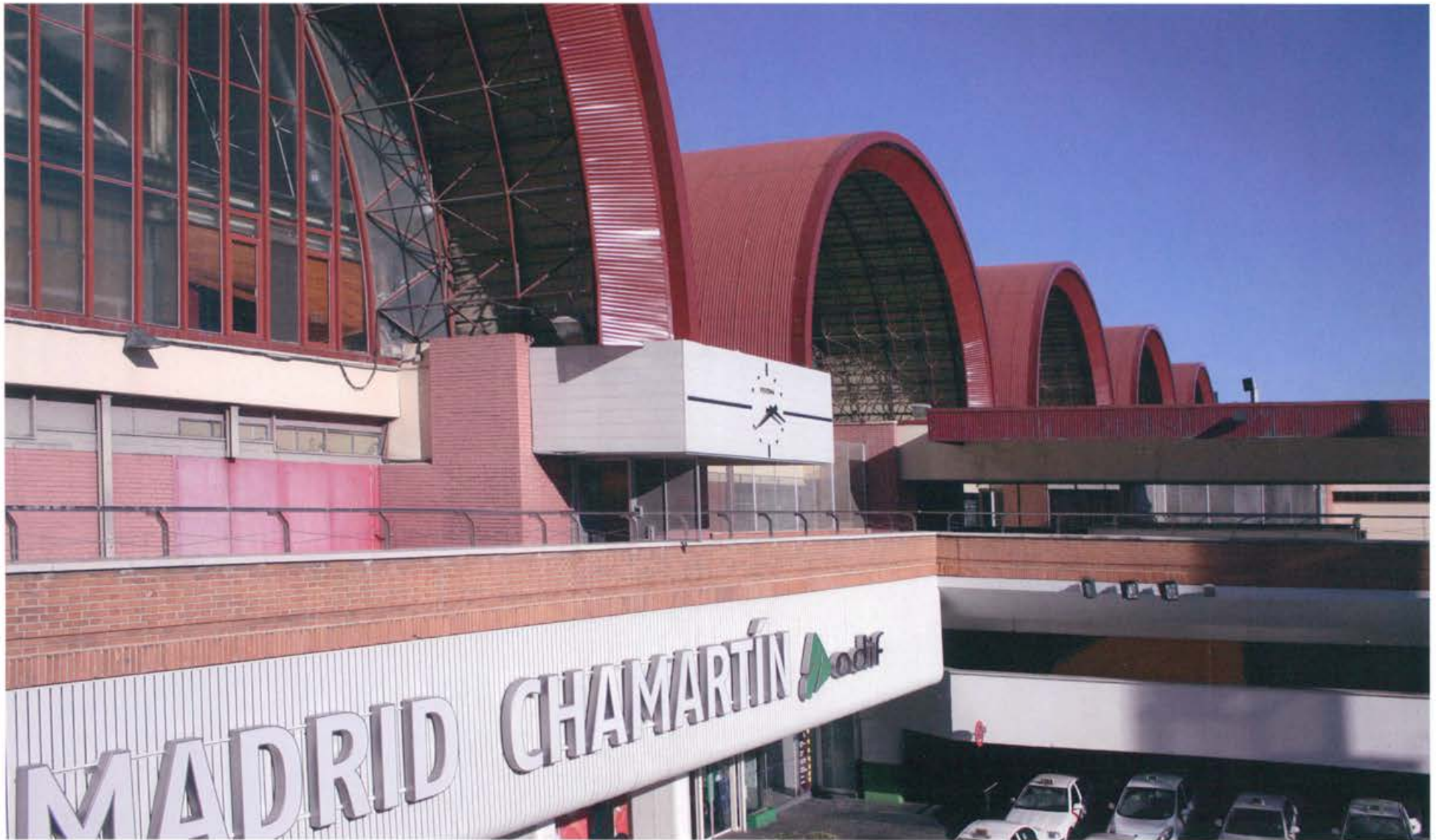
New Chamartín station and accesses
