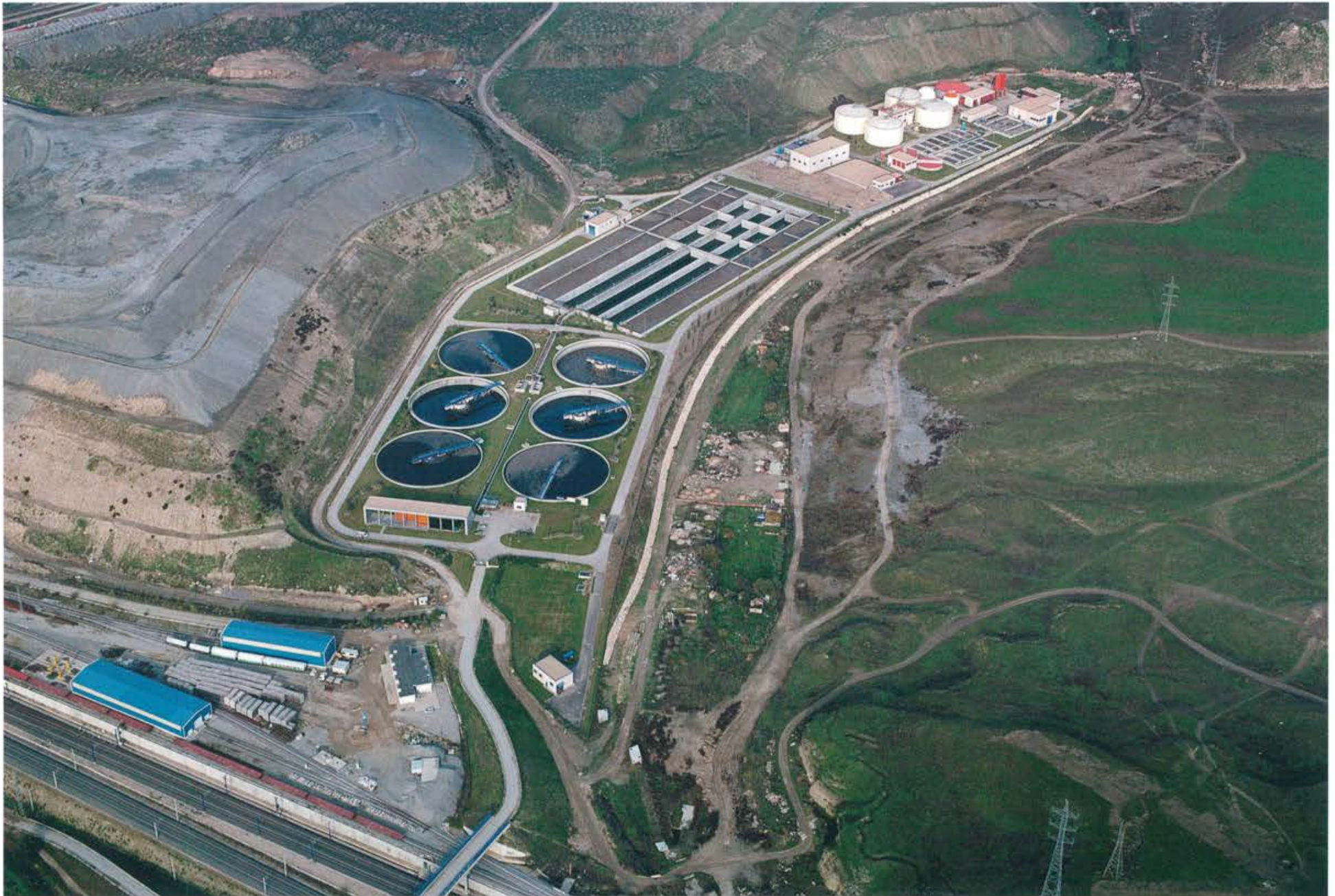
Gavia (Madrid) waste water treatment plant
