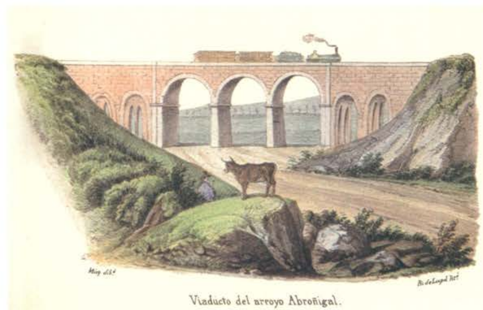
Railway viaduct on the Madrid - Aranjuez line over the Abroñigal brook [165:1]
