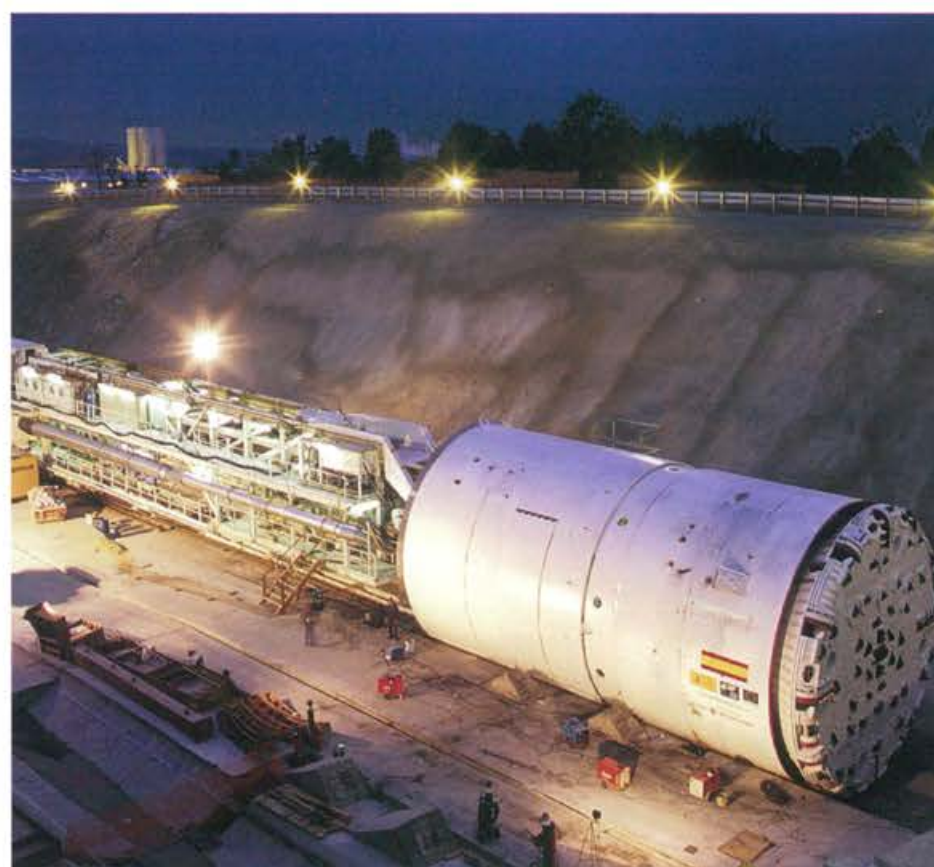
Guadarrama Tunnel, Southern Mouth. 2005
