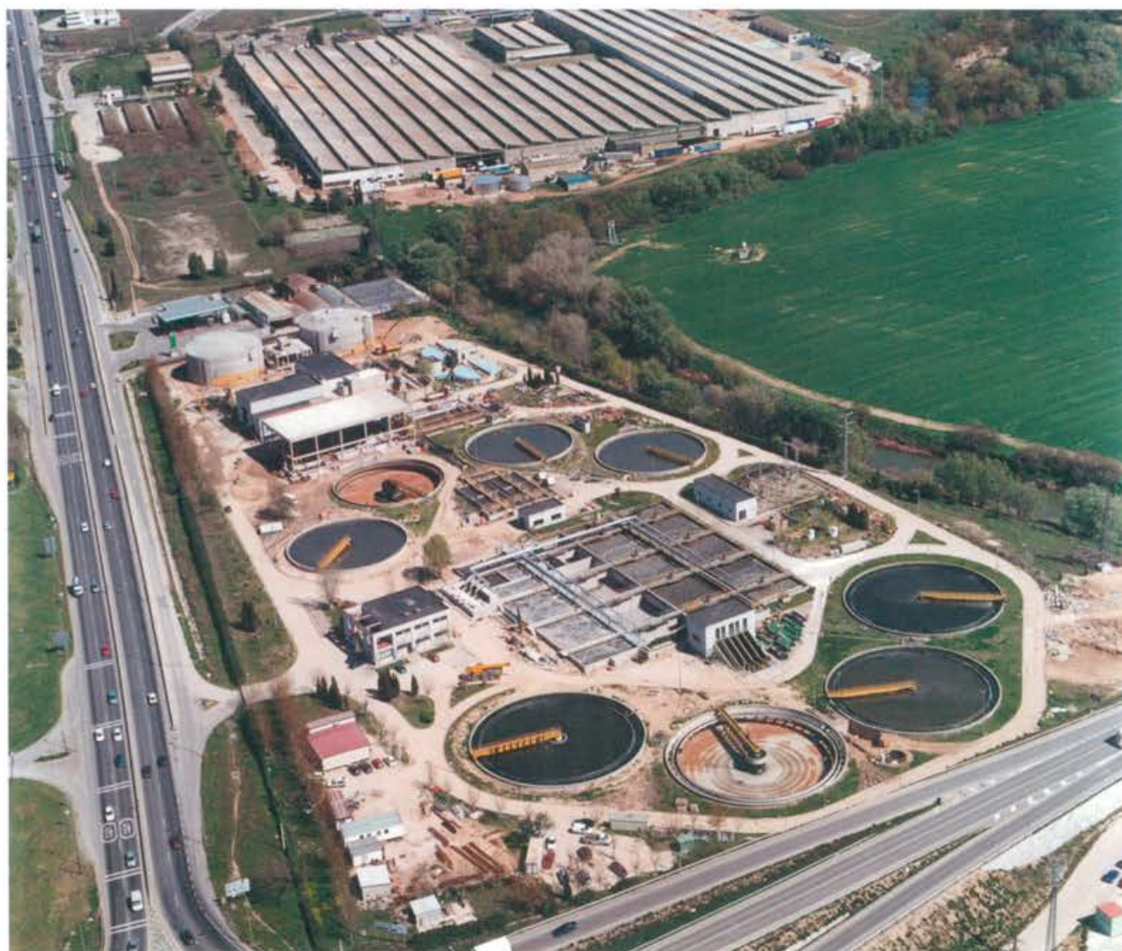
Alcalá Oeste industrial waste water treatment plant
