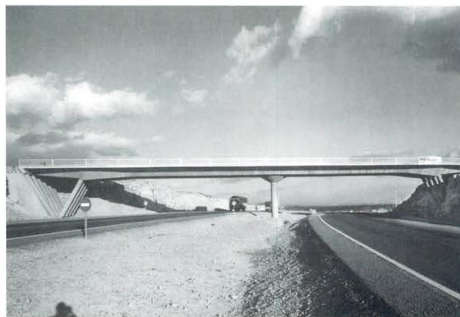
Bridge over the A6 road at Hoyo de Manzanares
