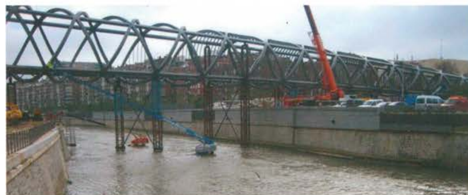
Arganzuela II footbridge. 2010
