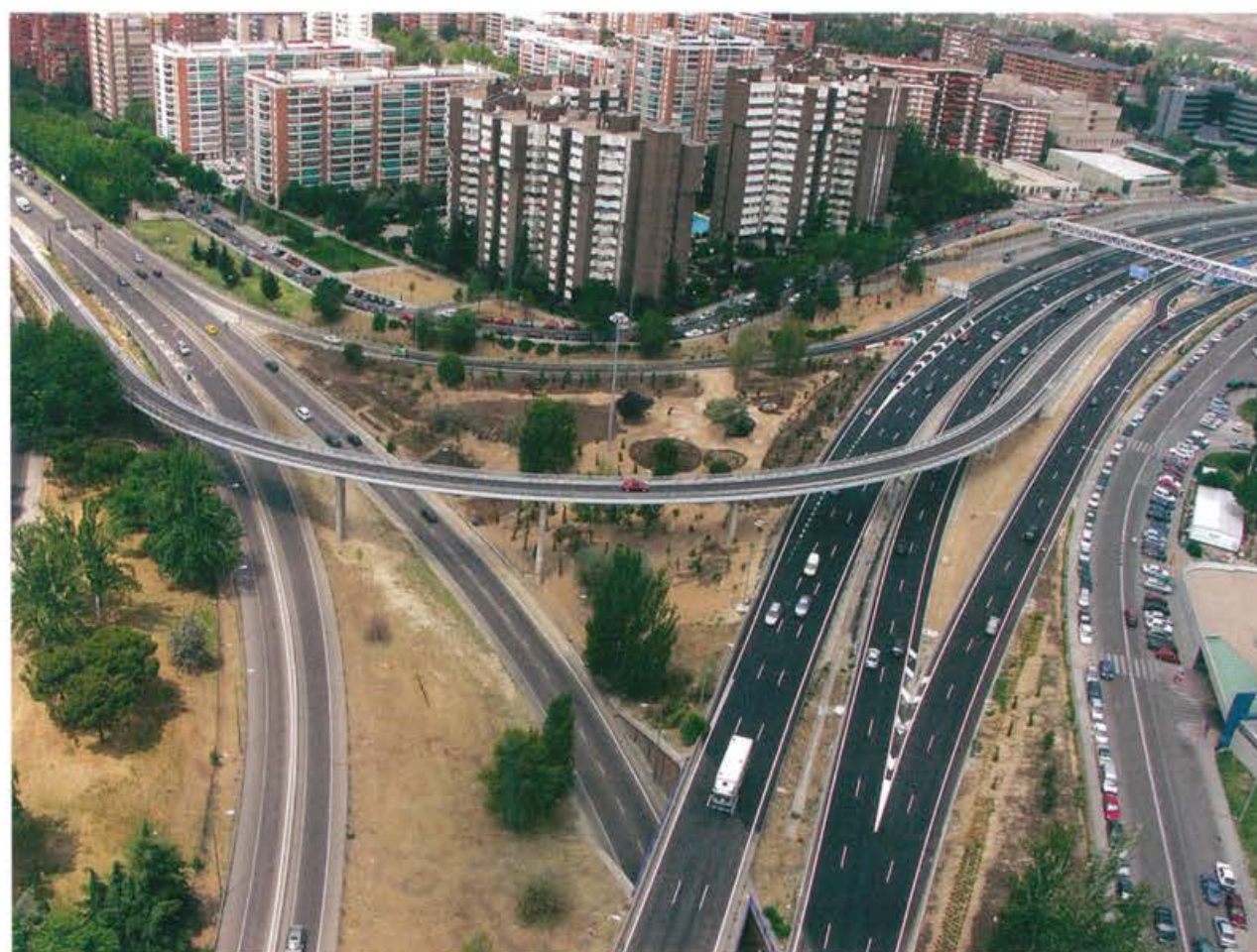
Northern completion of the M-30
