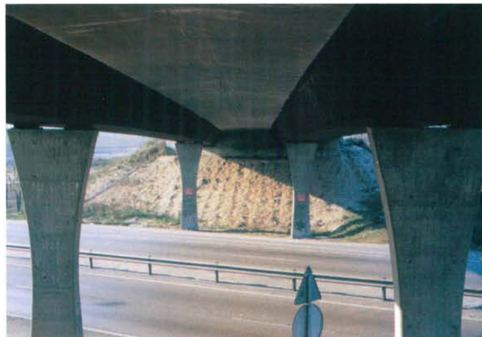
M-603 road over the M-607 highway at Colmenar Viejo Rui-Wamba, 1986
