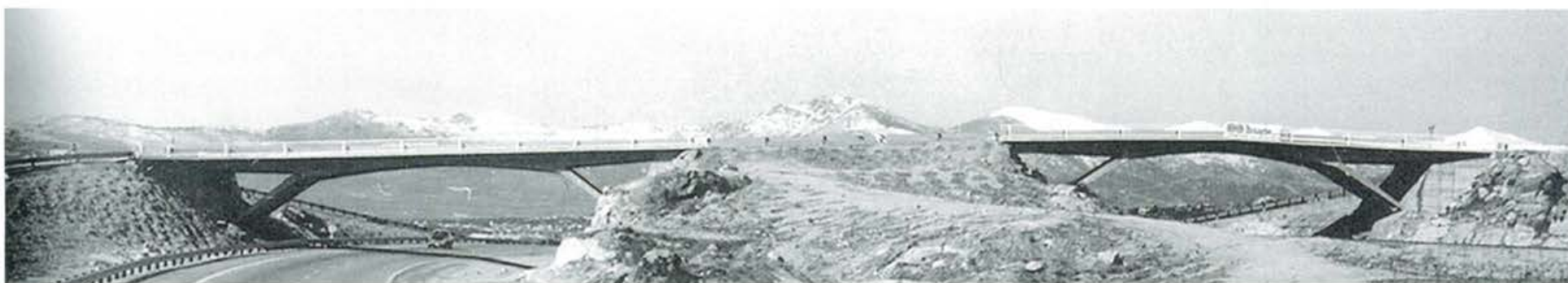
La Navata bridges over the A6
