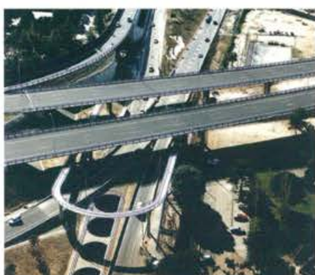
El Pardo junction footbridge, M-30 and M-40
