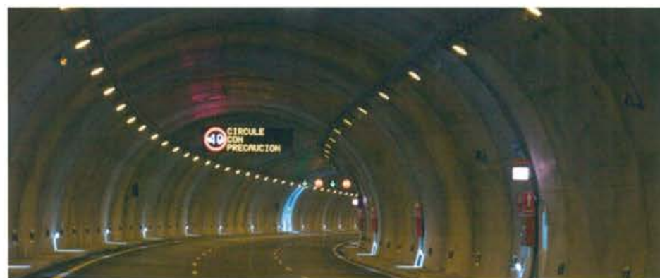
AP-6 motorway. Guadarrama tunnel. 2007
