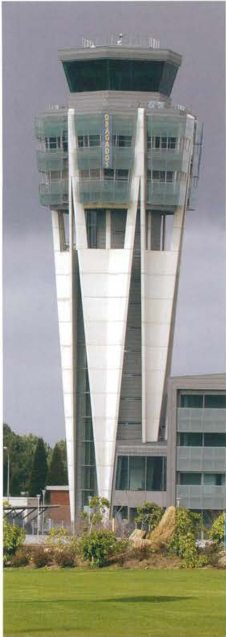
AENA control tower
