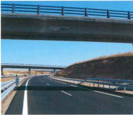
R-2 Radial Motorway (Madrid-Guadalajara)
