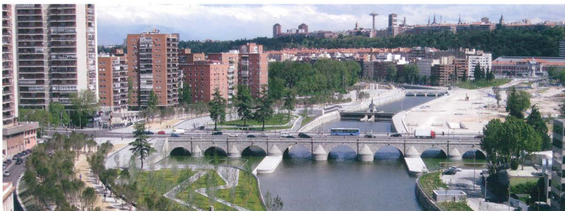
Madrid-Rio, historic area
