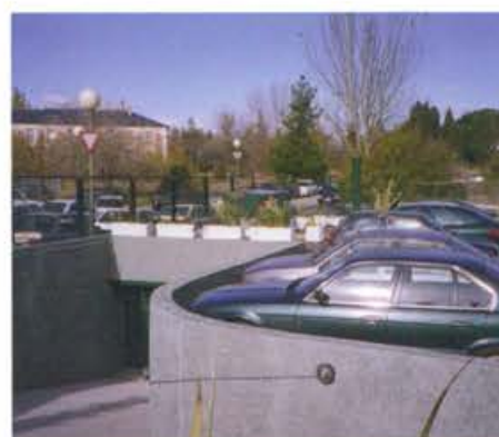
Calle Basauri car park
