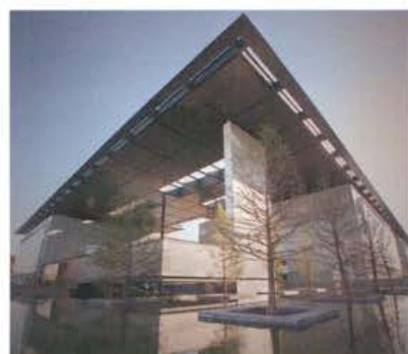
Telefónica Telecommunications City
