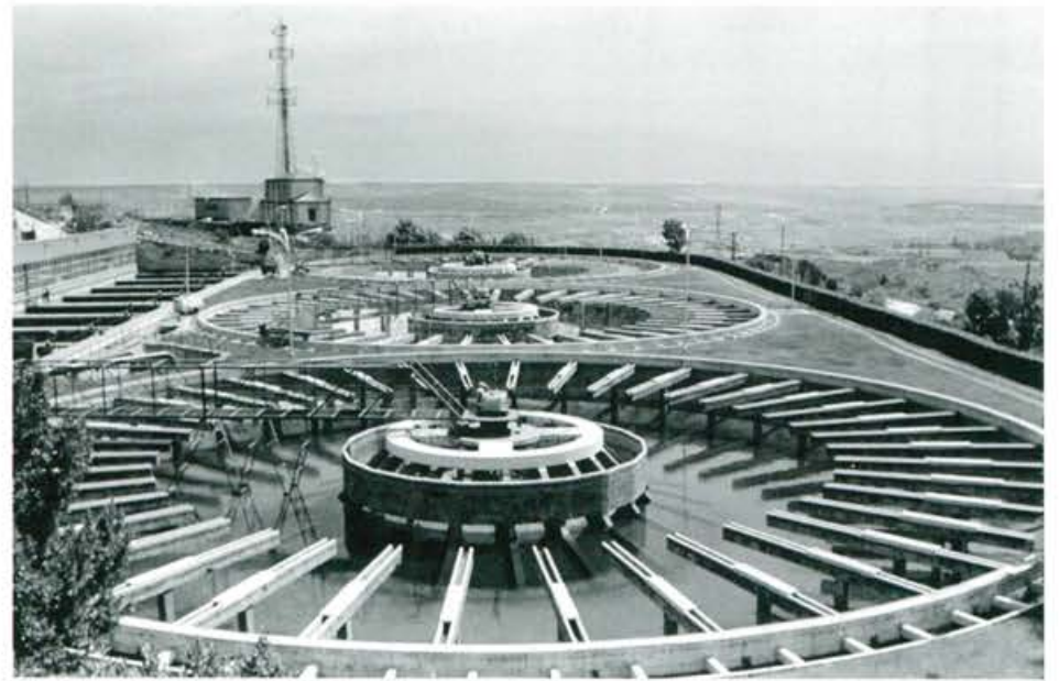
Torrelaguna water-treatment works [Photo: Antonio Sarabia]
