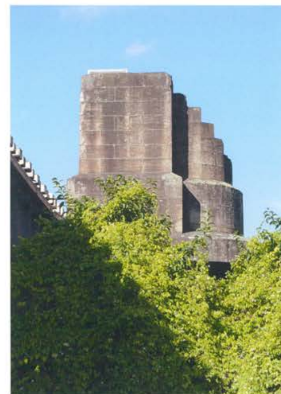
Menangle Railway Bridge, 1863
