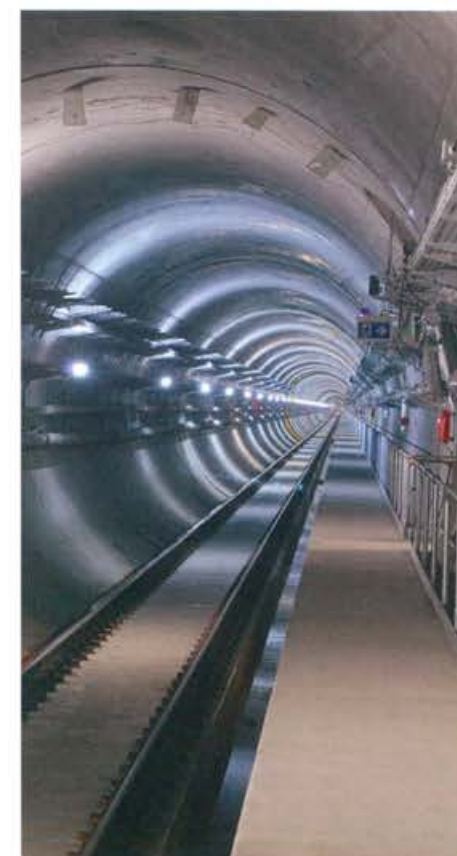
Epping to Chatswood Rail Line
