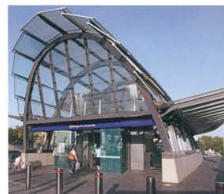
Epping to Chatswood Rail Line 14
