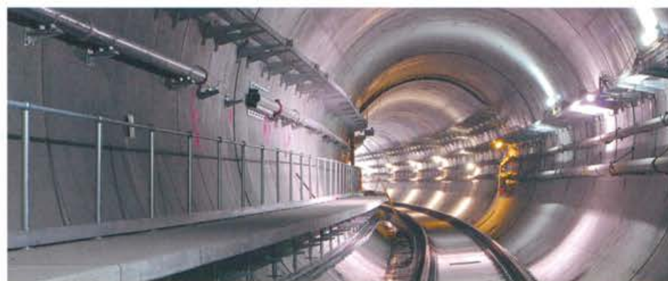
Epping to Chatswood Rail Line
