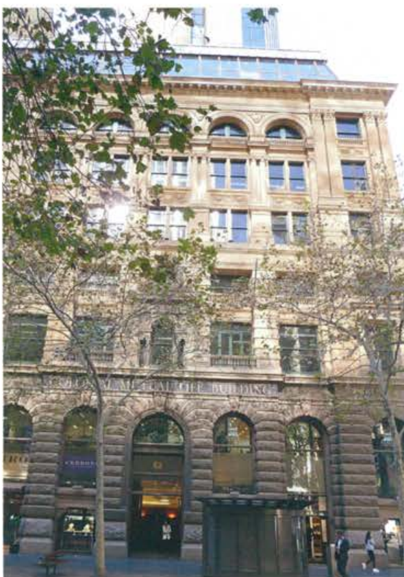
Colonial Mutual Life Building
