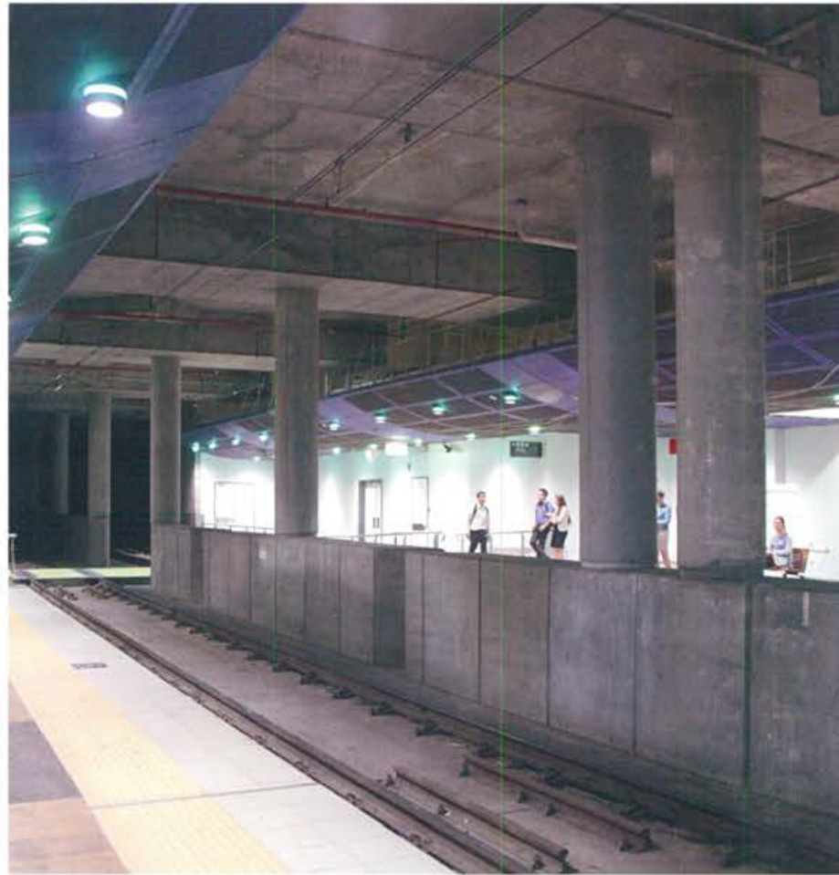
Light Rail en Central Station (1997)
