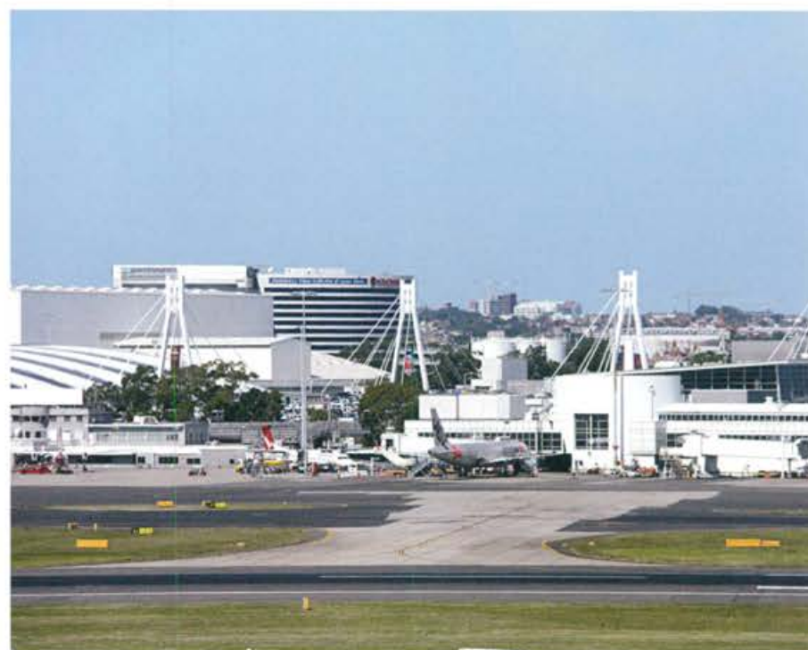
Sydney International Airport
