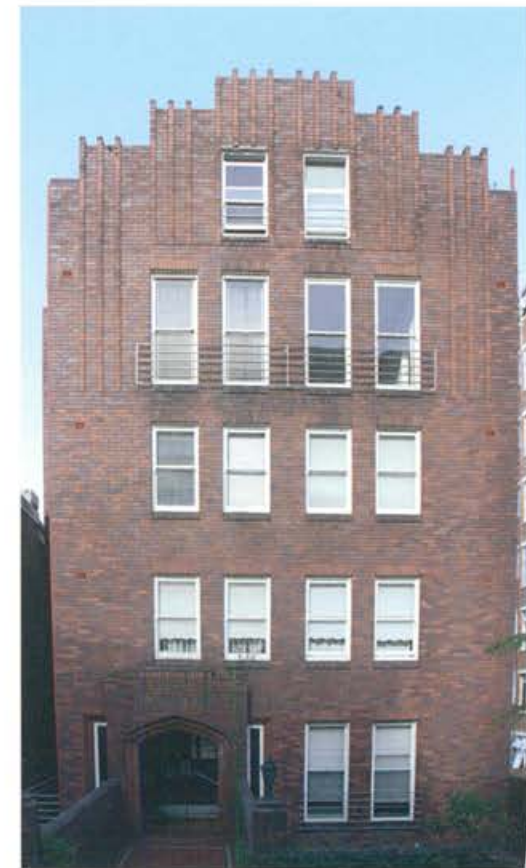
Edgewater Bldg., 6 Billyard Av, 1936
