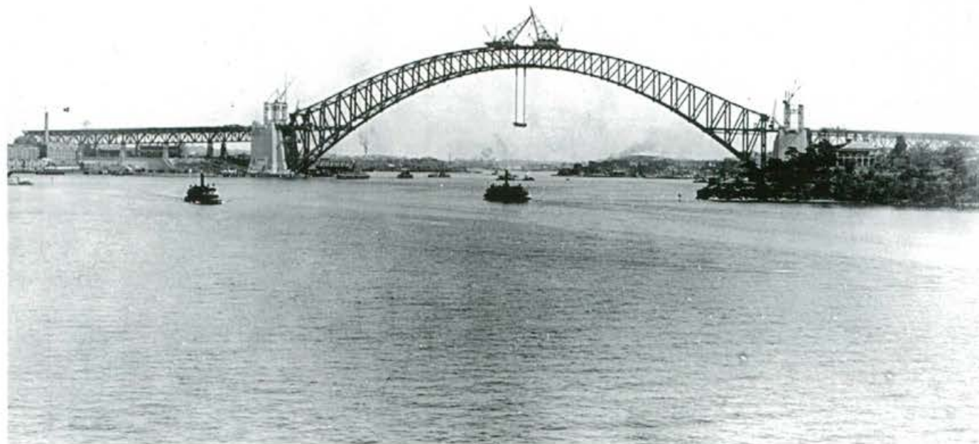
Looking west to the Harbour Bridge, road frames start construction, c. 1930. Courtesy of City of Sydney Archives. Graeme Andrews 'Working Harbour' Collection: 79788
