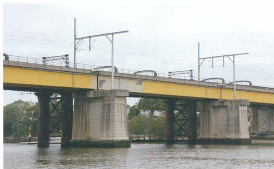
Meadowbank Rail Bridge, 1885
