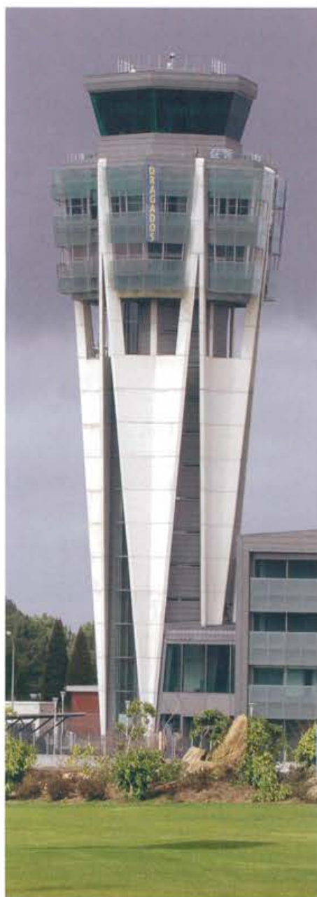
Torre Control Aena
