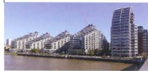
Ascensis Tower & Comodore House
