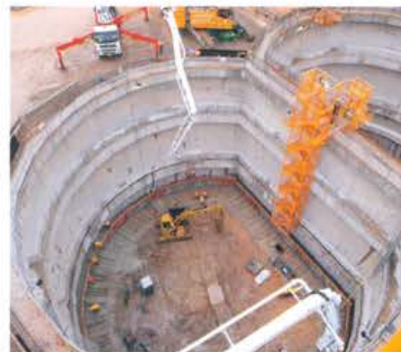
West Connex tunnel, Sidney, Australia
