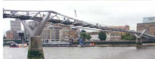
2002 Millennium Bridge 3, colgante, acero City: Queenhithe / Bankside
