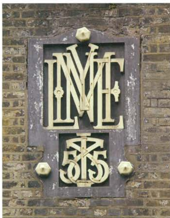
Stoke Newington Pumping Station, 1852
