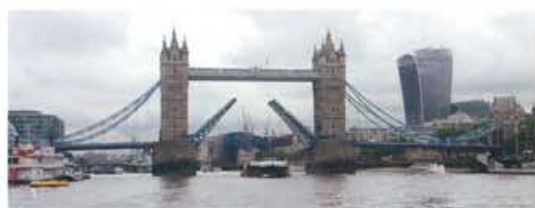
1894 Tower Bridge 3, basculante, acero Tower Hamlets / Southwark
