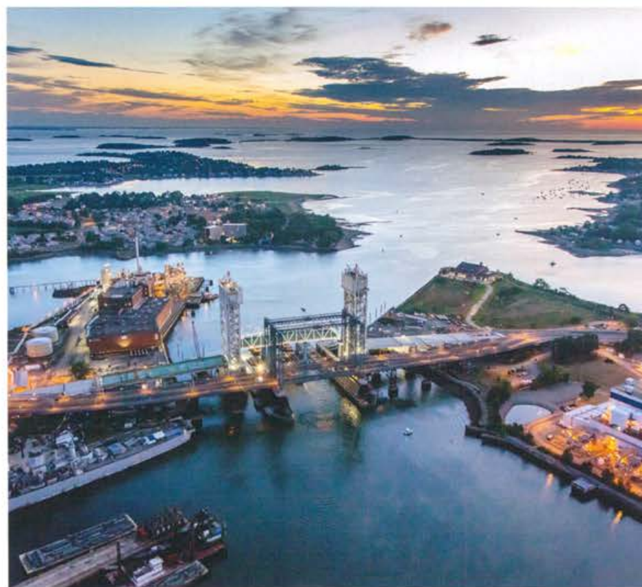
Mip Aerial Fore River Bridge
