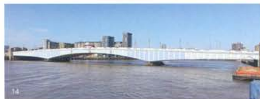
1938 Wandsworth Bridge 3, viga continua, acero Fulham / Wandsworth
