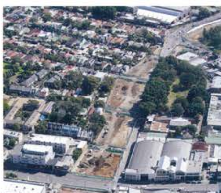
West Connex, Local Roads, Sidney, Australia
