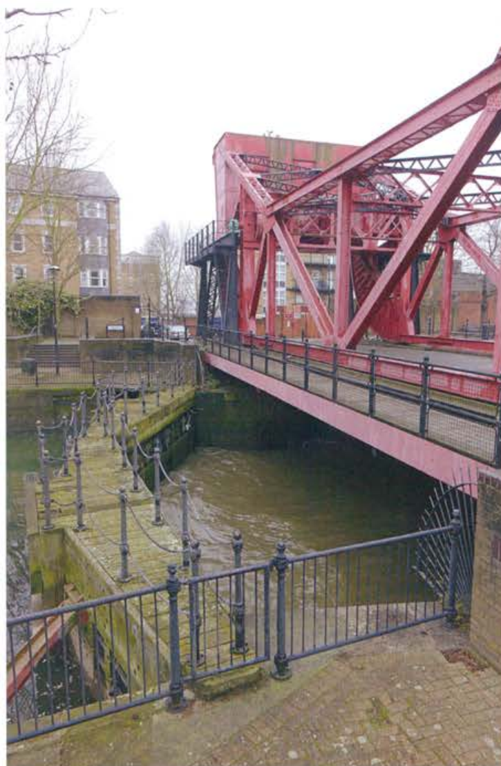
Surrey Docks -Old Salt Quay Bridge Greenland Docks-Swing Bridge
