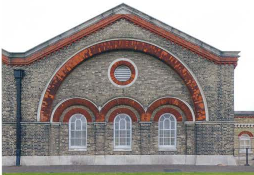
Crossness Pumping Station
