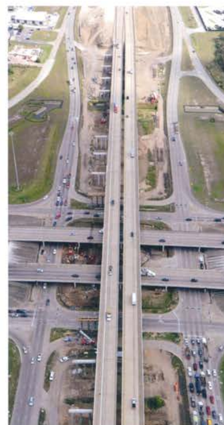
Sam Houston Tollway SE Widening, West of SH 288 to West of Wayside Dr.
