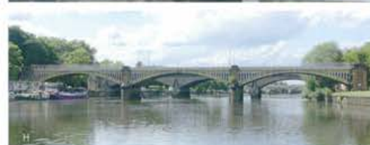
1848 Richmond Railway Bridge 4, arco, hierro St Margaret / Richmond
