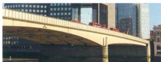
1973 (1831, 1209, 50) London Bridge 3, viga continua, hormigón City: Monument / Southwark
