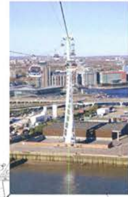
Emirates Cable Car
