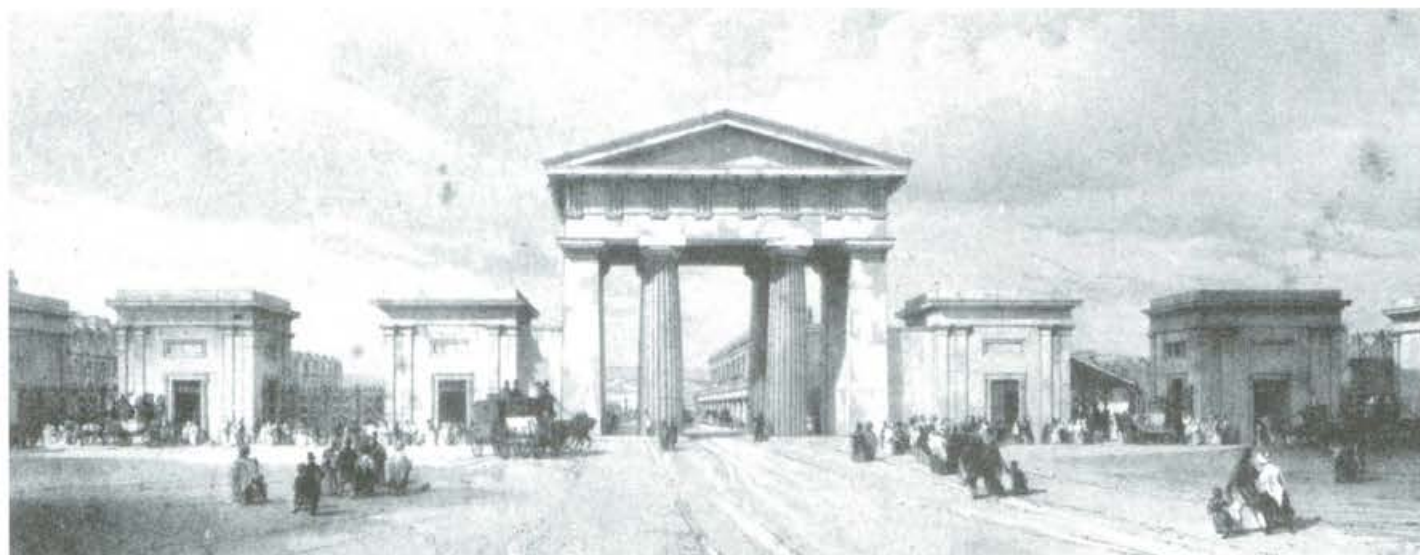
Old Euston Station - pórtico, 1837 [88:fig17]
