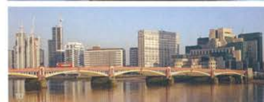
1905 Vauxhall Bridge 5, arco, acero Pimlico / Vauxhall
