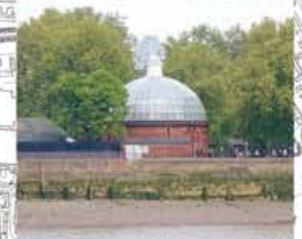
Greenwich Footway Tunnel
