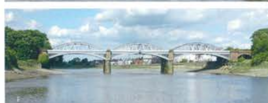
1895 & 1849 Barnes Rv Bridge & Footbridge 3, bowstring, hierro Chiswick / Barnes
