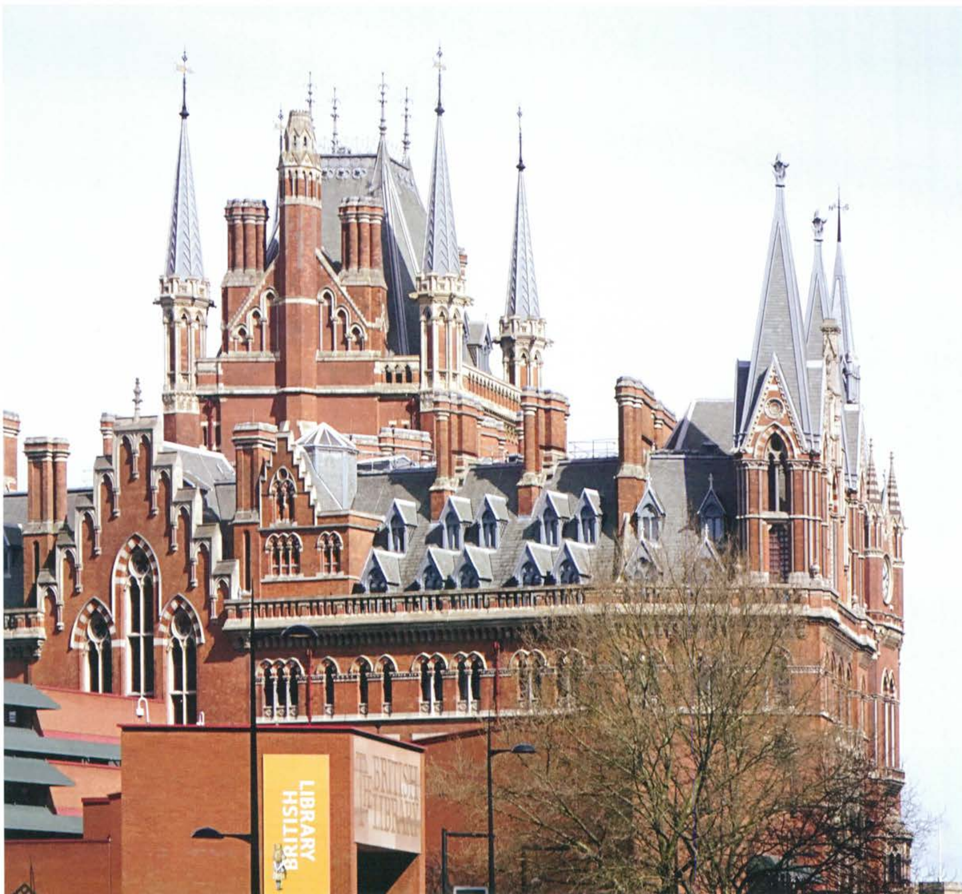
St Pancras Station - torreones
