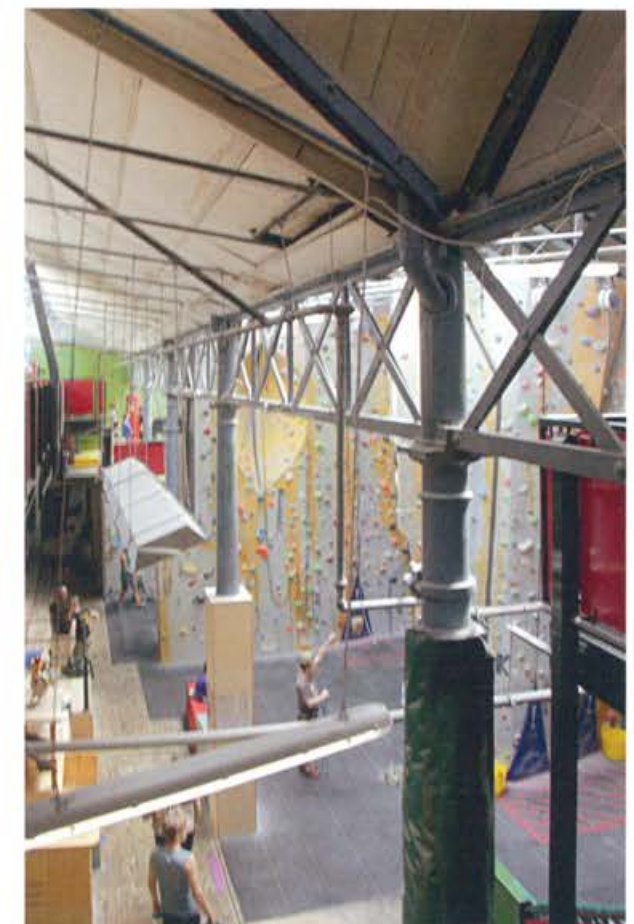
Stoke Newington West Reservoir Centre Stoke Newington Pumping Station - Castle Climbing Centre
