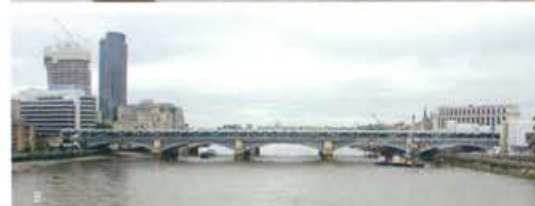
1886 (1864) Blackfriars Railway Bridge 5, arco, hierro City: Blackfriars / Southwark
