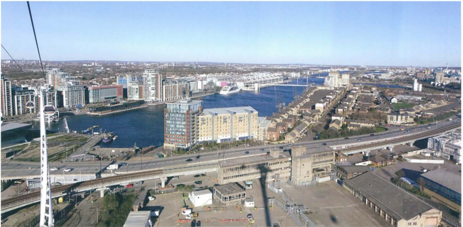
District Light Rail
