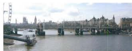
2002-1864 (1845) Hungerford & Golden Jubilee Br 7, cable-stayed, steel Westminster / South Bank
