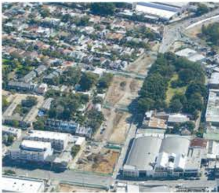
West Connex, Local Roads, Sydney, Australia
