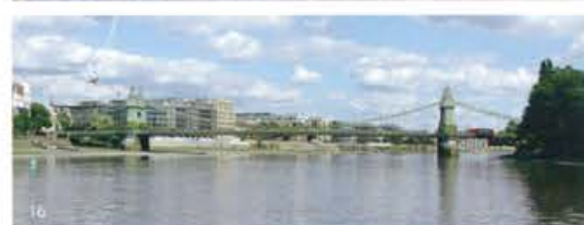
1887 (1827) Hammersmith Bridge 3, pendant, iron Hammersmith / Castelnau
