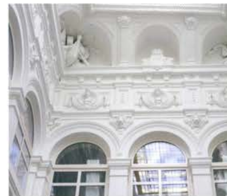
Custom headquarters rehabilitation, Bilbao
