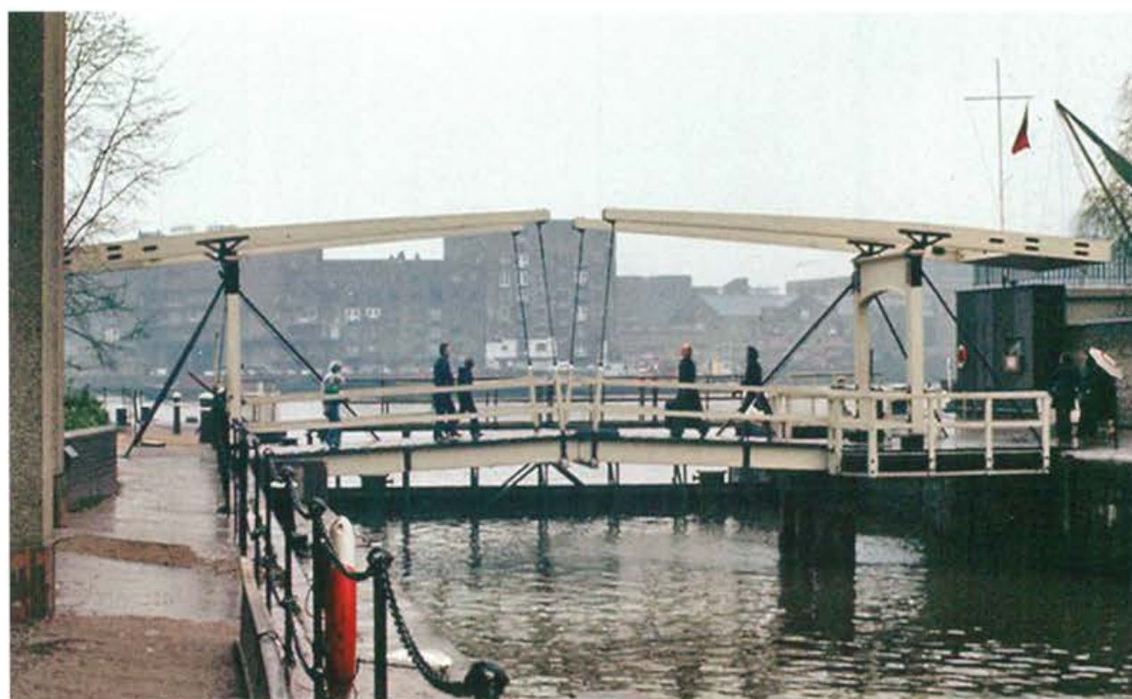
Western dock drawbridge in 1976
