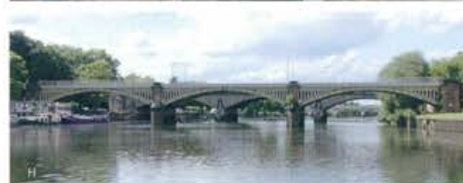
1848 Richmond Railway Bridge 4, arch, iron St Margaret / Richmond
