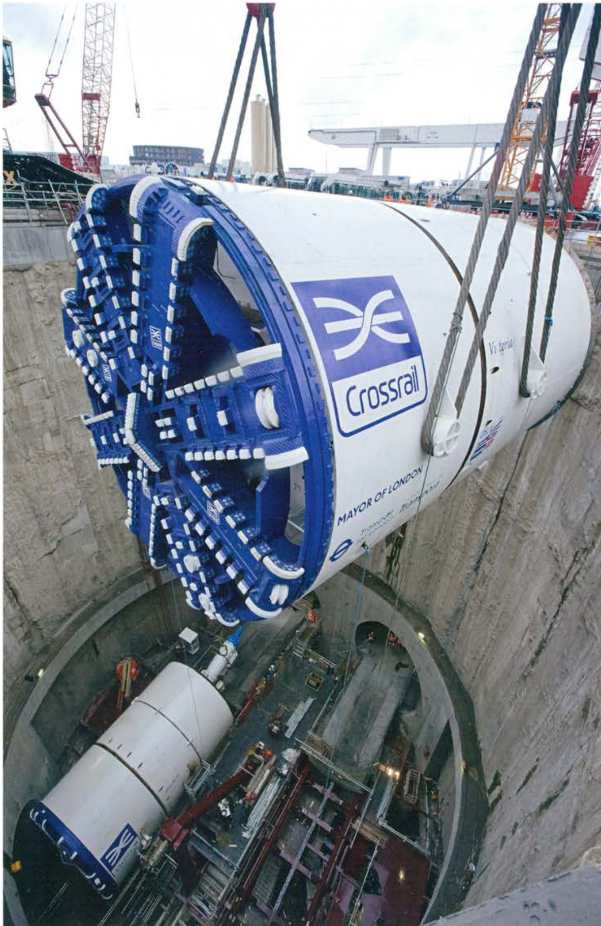
Tunnel boring machine and Crossrail tunnel
