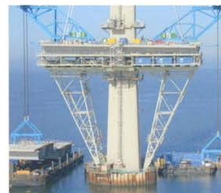
Highway Windsor Essex Parkway, Ontario, Canada. 2015
