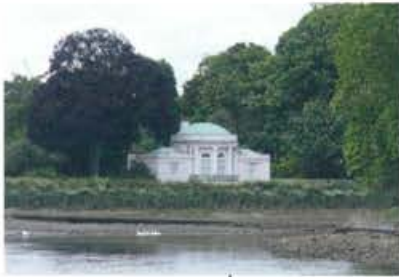
Pavilion in Syon Park
