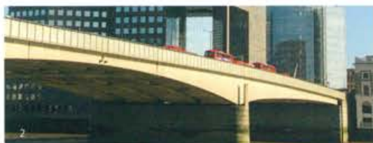
1973 (1831, 1209, 50) London Bridge 3, continuous beam, concrete City: Monument / Southwark
