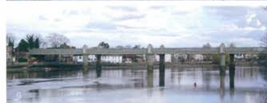
1869 Kew Railway Bridge 5, lattice beam, iron Gunnersbury / Kew Gardens
