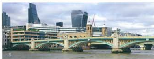
1921 (1819) Southwark Bridge 5, arch, steel City: Queen Street / Bankside
