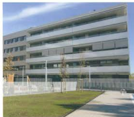
San Cugat del Vallés Housing, Barcelona
