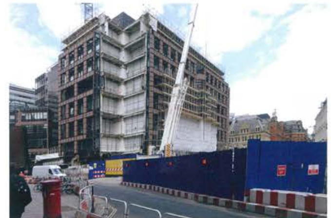
Crossrail Broadgate Entrance - construction
