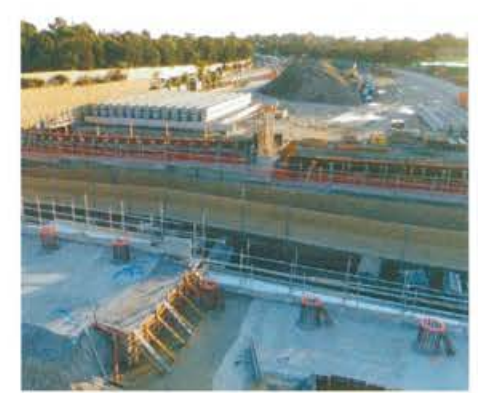
West Connex, Sydney, Australia
