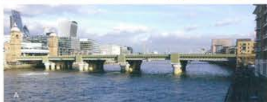
1866 Cannon Street Railway Bridge 5, beam, iron City: Cannon St / Southwark
