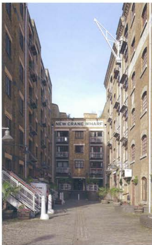
New Crane Wharf
