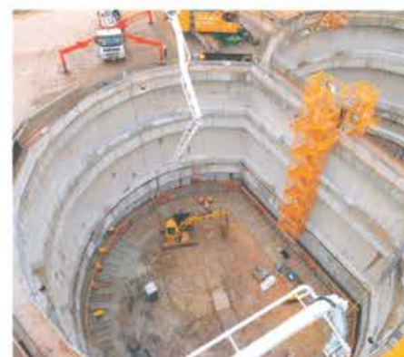
West Connex tunnel, Sydney, Australia
