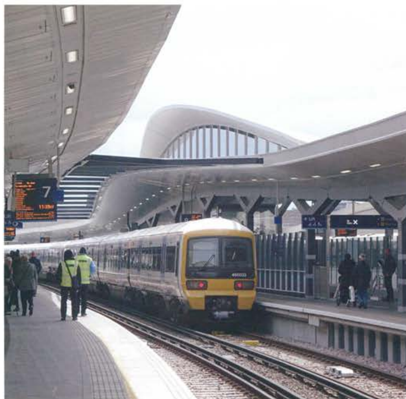
London Bridge Station
