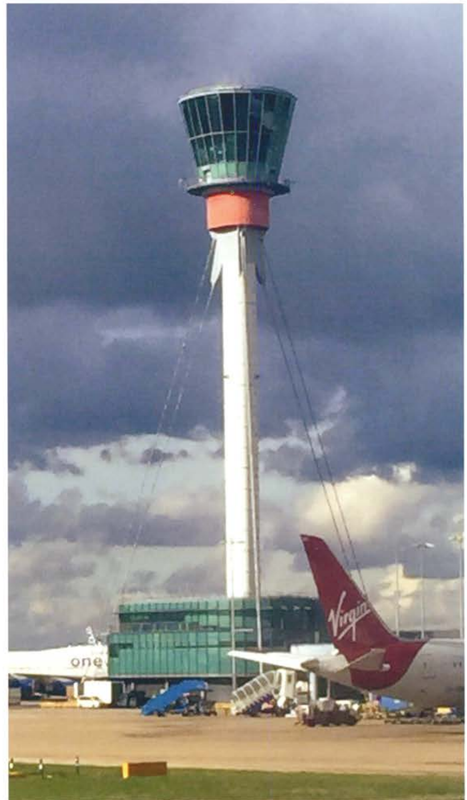
Control tower. Heathrow Airport T5
