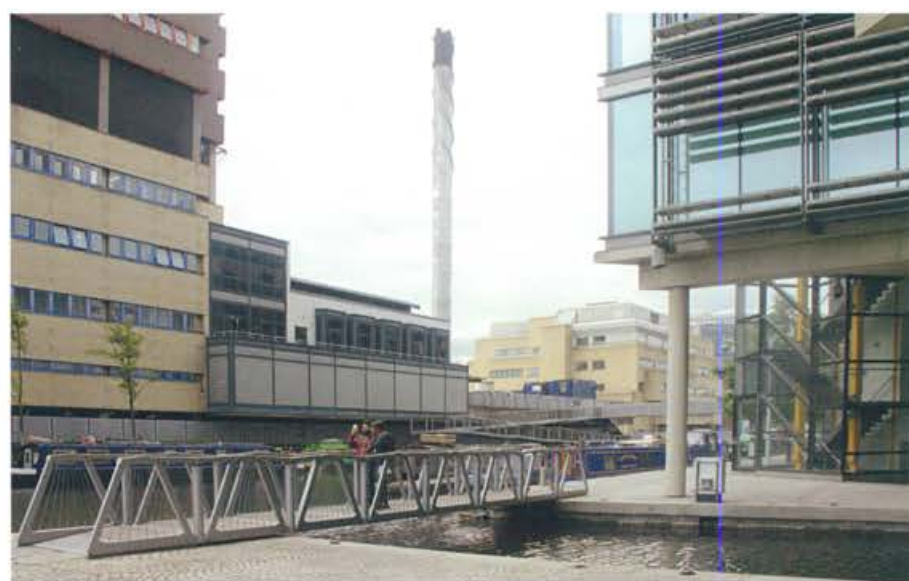
Bridge-Paddington Basin (Heatherwick studio & Anthony Hunts) - The structure opens by means of a series of hydraulic cylinders arranged on the beam platform of the bridge; as it rolls up, each of its eight segments rises simultaneously, until the two ends touch each other forming an octagon. 21
