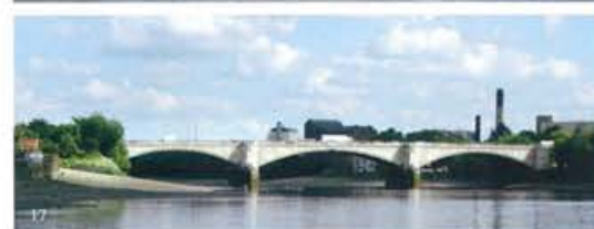
1933 Chiswick Bridge 3, arch, stone Chiswick / Mortlake
