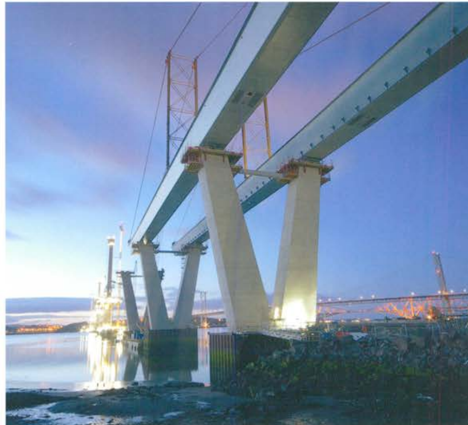
New Bridge Queensferry Crossing, Scotland
