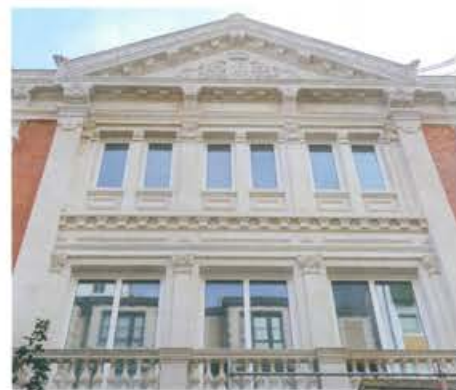
Custom headquarters rehabilitation, Bilbao
