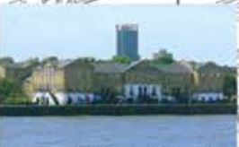
Trace Houses, Rotherhithe St
