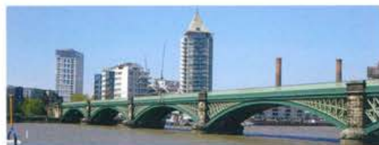
1863 Battersea Railway Bridge 5, arch, iron Imperial Wharf / Clapham Junct
