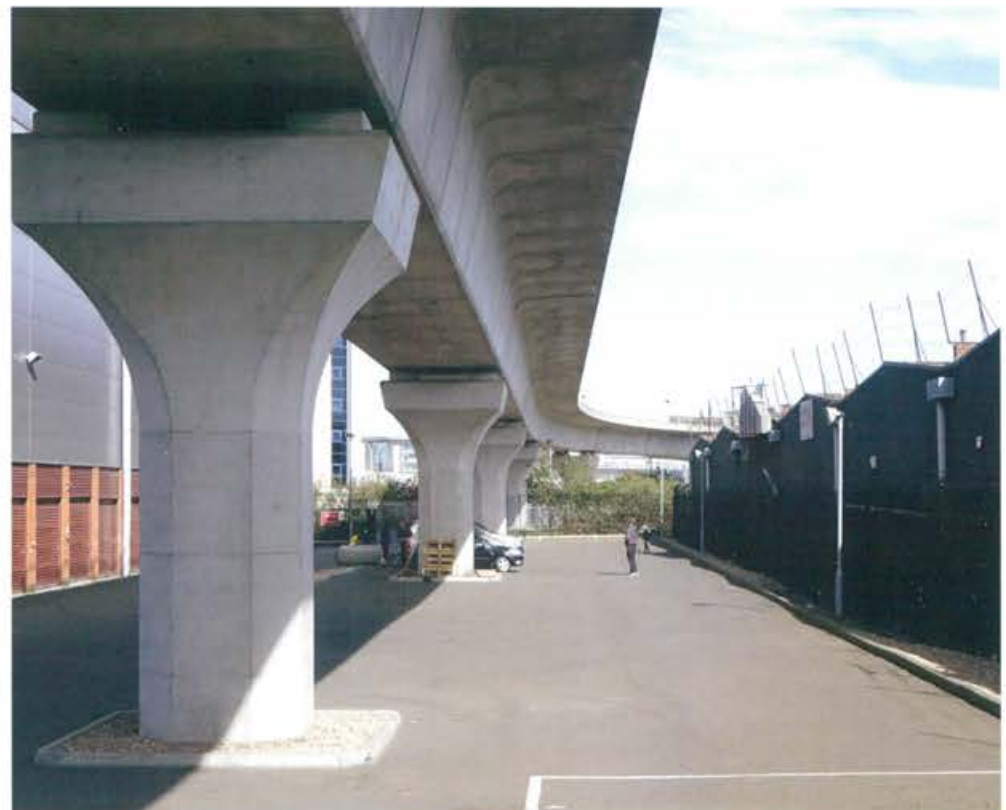
District Light Rail
