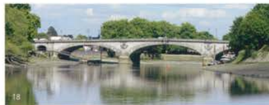
1903 Kew Bridge 3, arch, stone Brentford / Kew
