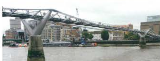
2002 Millennium Bridge 3, pendant, steel City: Queenhithe / Bankside
