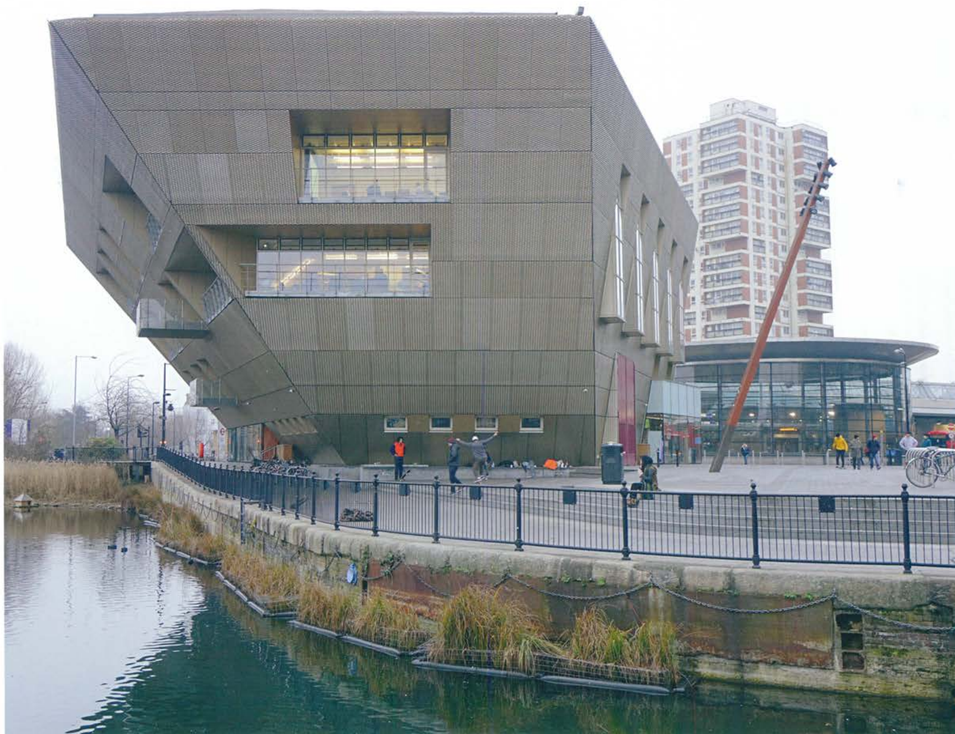
Canada Water-Jubilee Line Station
