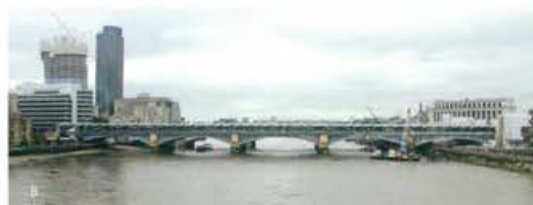
1886 (1864) Blackfriars Railway Bridge 5, arch, iron City: Blackfriars / Southwark
