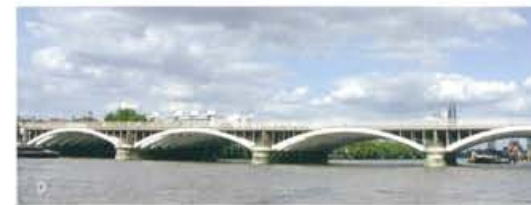
1967 (1859) Grosvenor Railway Bridge 5, arch, iron Westminster / Wandsworth
