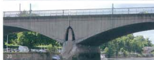
1933 Twickenham Bridge 3, arch, concrete St Margaret / Richmond
