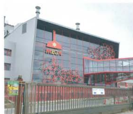
Mega building rehabilitation, Galicia
