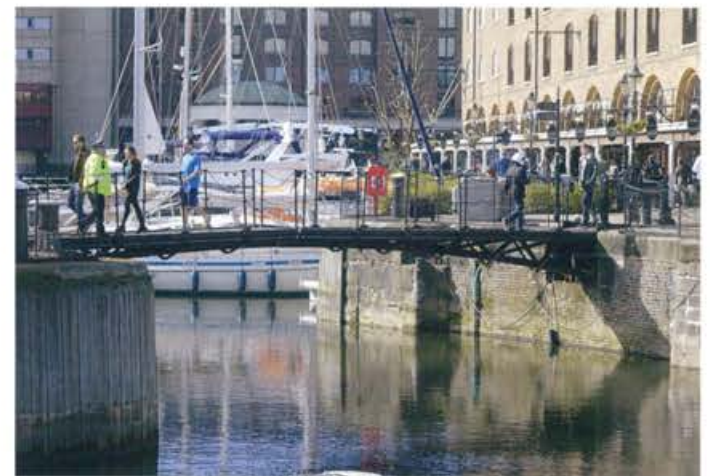
Eastern dock retractable bridge
