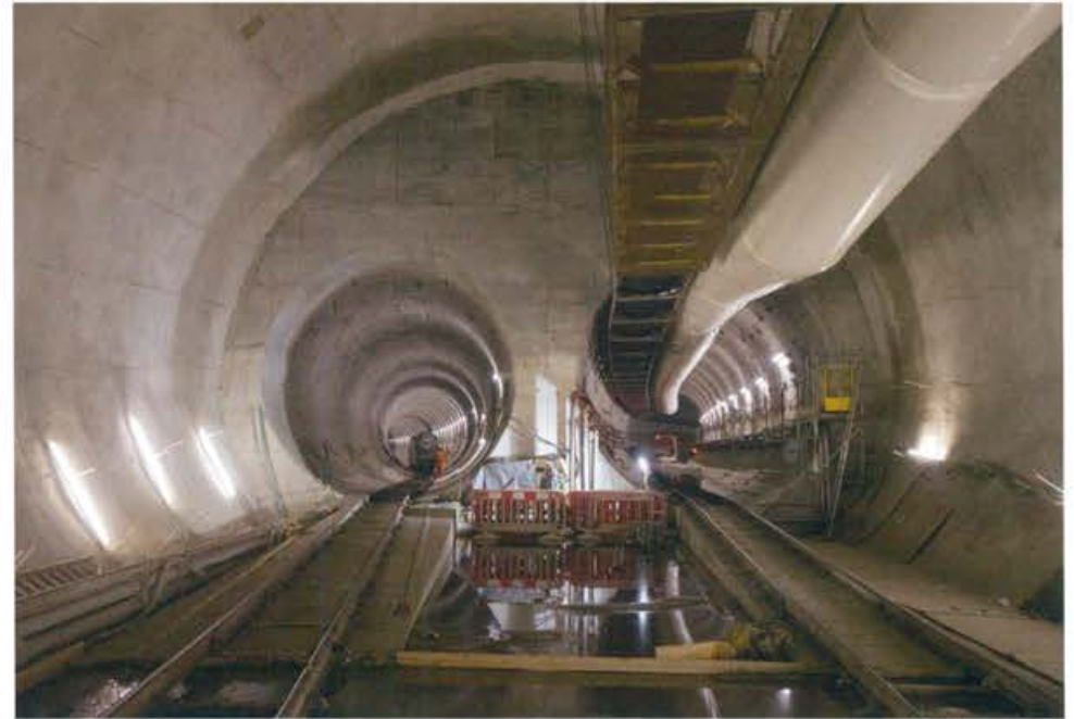
Double Crossrail tunnel
