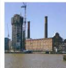
Chelsea Power Station
