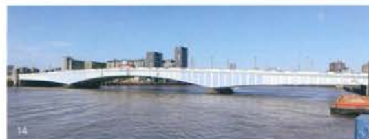
1938 Wandsworth Bridge 3, continuous beam, steel Fulham / Wandsworth
