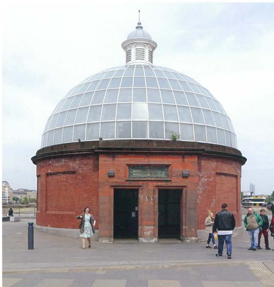
Greenwich Footway Tunnel, LCC, 1902
