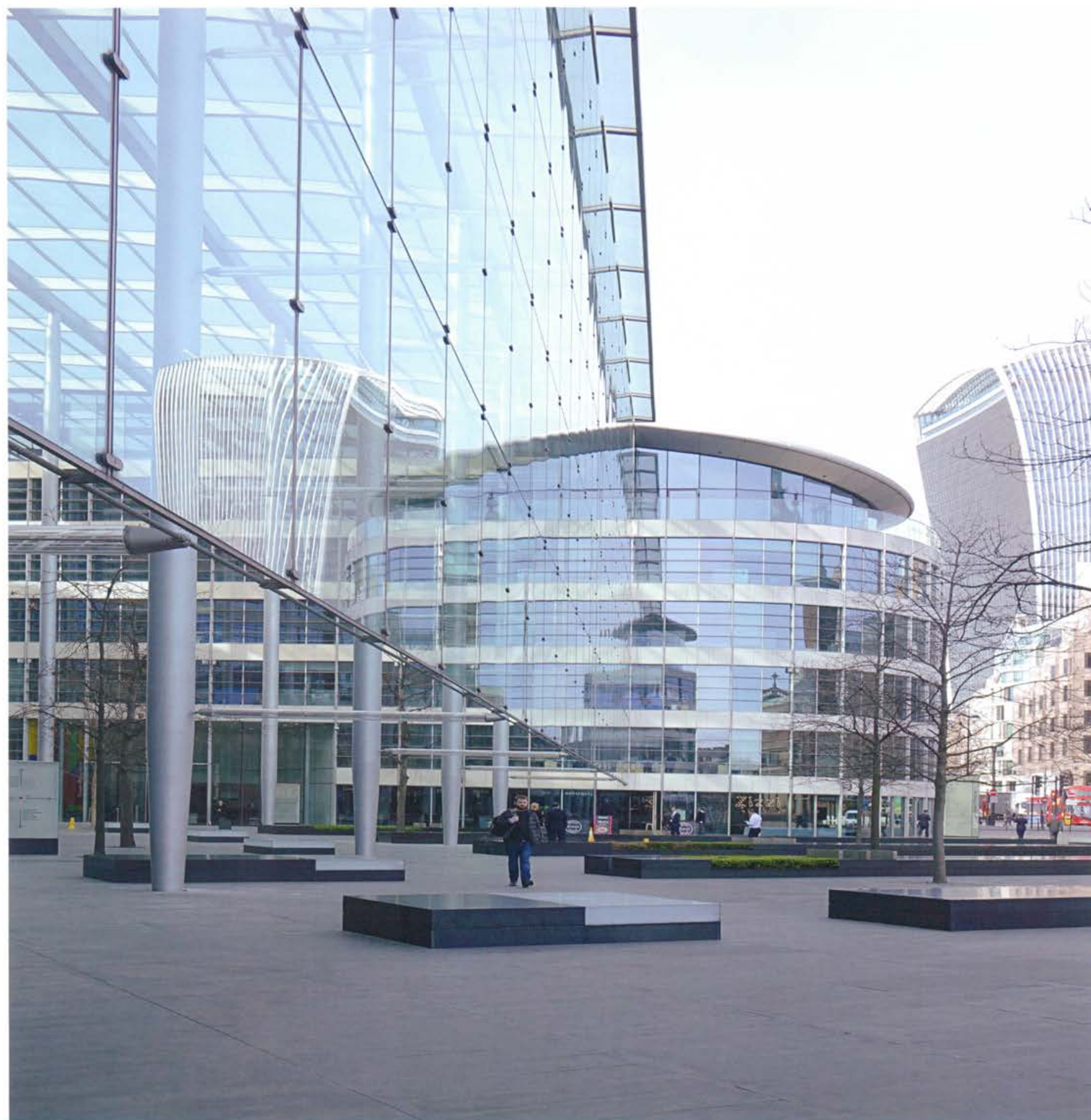
Tower Place (Foster, 2002)
