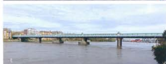
1889 (1729) Fulham Rv Br & Footbridge 7, lattice beam, iron Putney Bridge / East Putney
