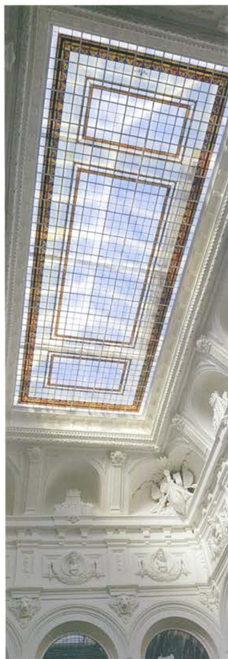
Custom headquarters rehabilitation, Bilbao
