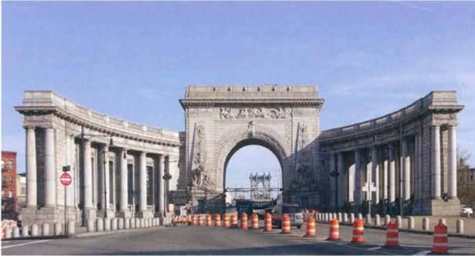
Urban scale of the Manhattan Bridge east access gate
