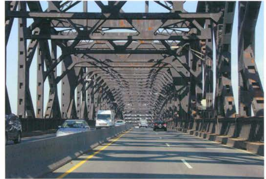
Entrances to the tunnel with the General Pulaski Skyway (Hugh L. Sloan, 1932)
