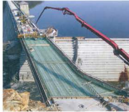
Croton Falls Dam, Westchester County, NY. 2012
