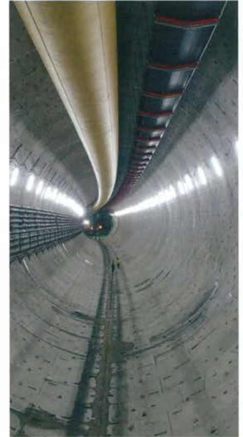
Alaskan Way Tunnel, Seattle
