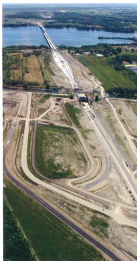
Soulanges Tunnel, sector 1. 2012
