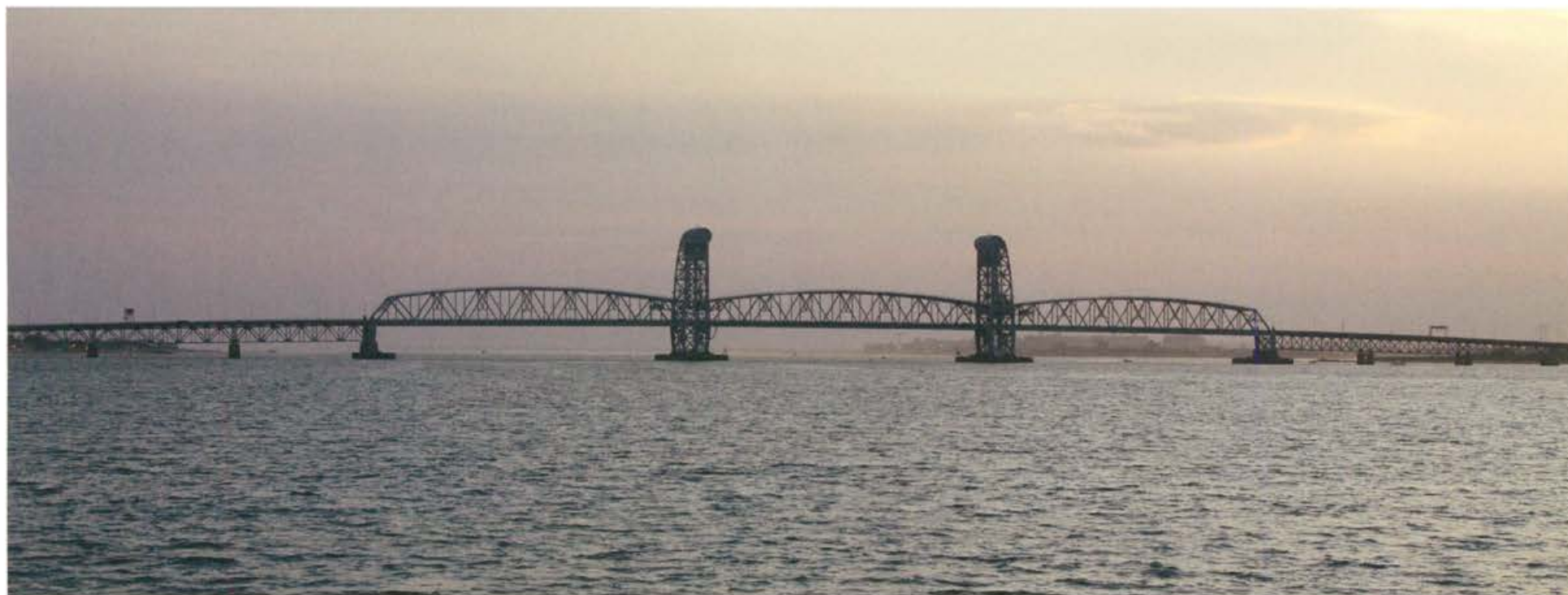
Marine Parkway Bridge
