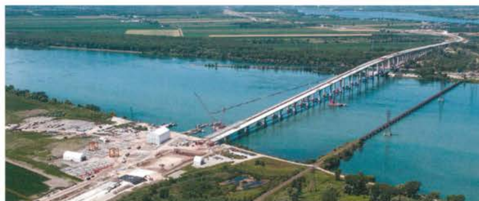
Beauharnois, Bridge sector 4. 2012
