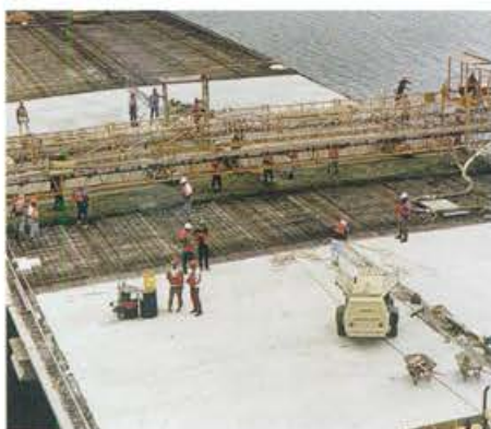
Teodoro Moscoso Bridge, Puerto Rico
