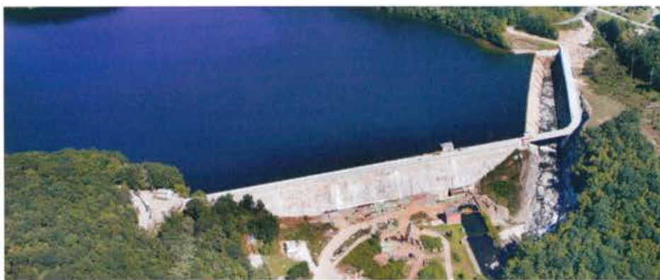
Croton Falls Dam, Westchester County, New York. 2012
