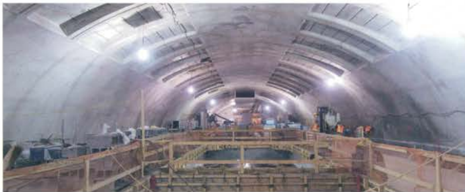
Second Avenue Subway
