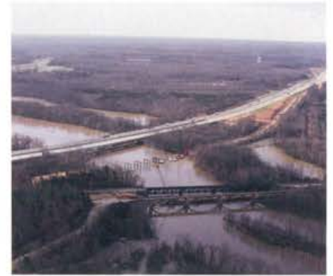
Yadkin River Bridge 2013
