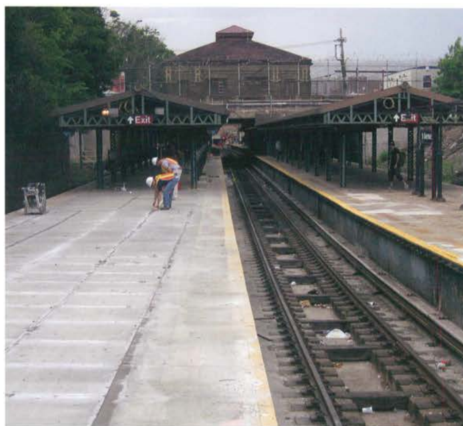
Brooklyn Subway. Refurbishing 5 stations, New York, USA. 2010
