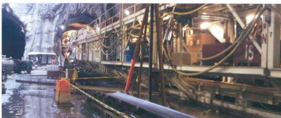
Second Avenue Subway
