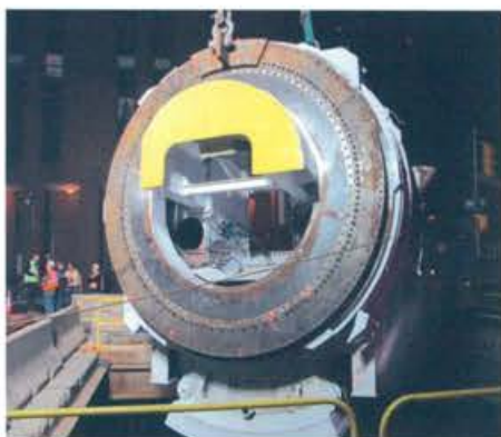
Second Avenue Subway
