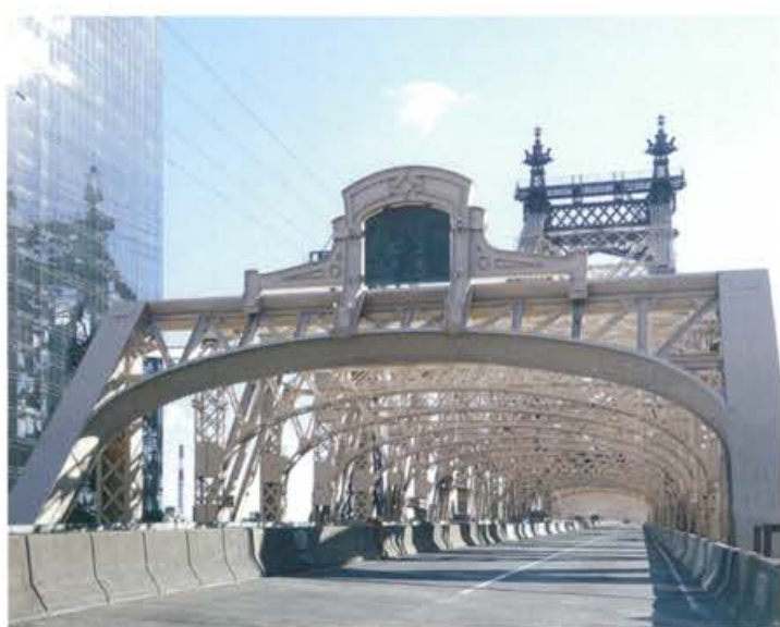
Queensboro Bridge (Gustav Lindenthal, Leffert L. Buck, 1909)
