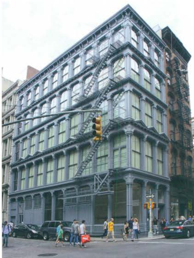
Cast-iron architecture in Lower Manhattan
