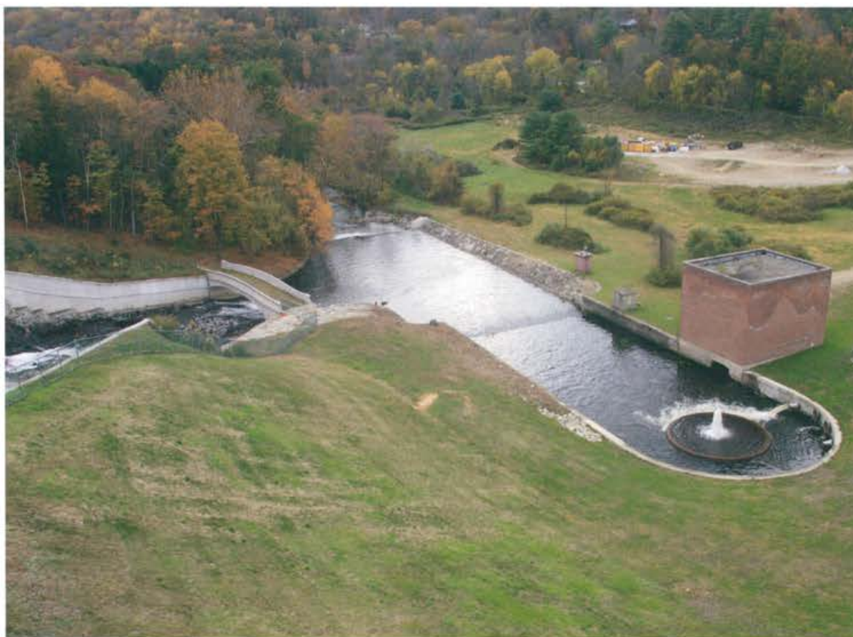
Croton Falls Dam (1911)
