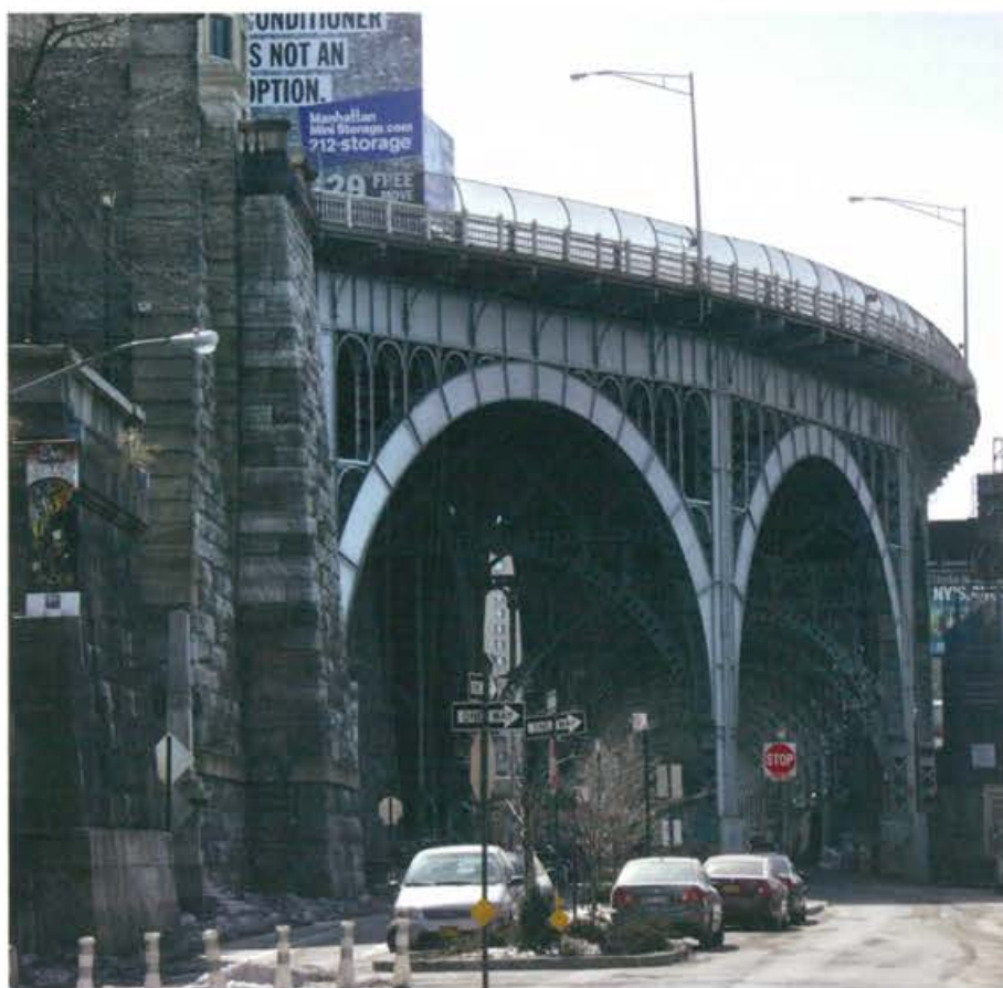
Riverside Drive Viaduct
