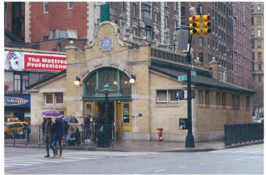
Control House North (Gruzen Samton and Richard Dattner & Partners, Architects, 2002)
