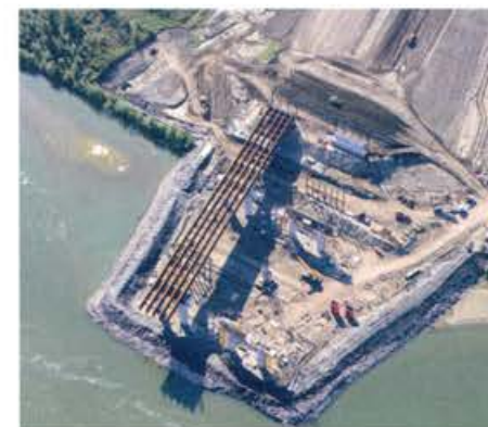
NEAH Construction of the bridge over Saskatchewan River
