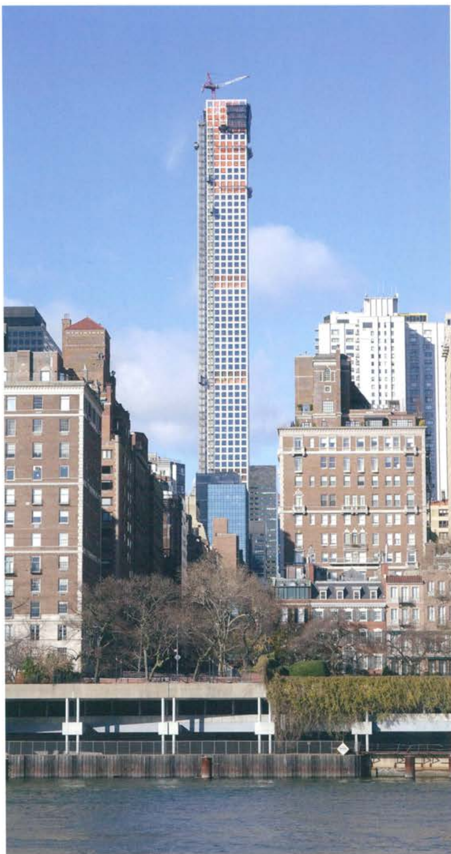
Park Avenue and 57th St. (under construction)
