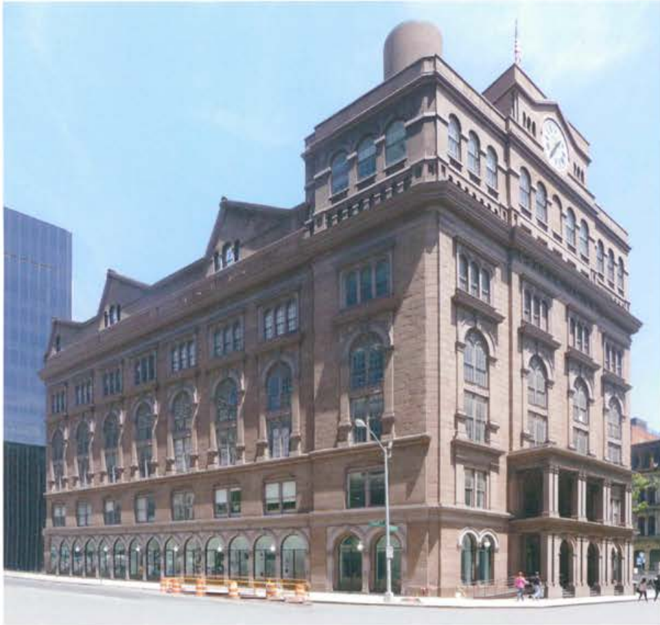
Cooper Union Bldg. (Cooper & Peterson, 1858)
