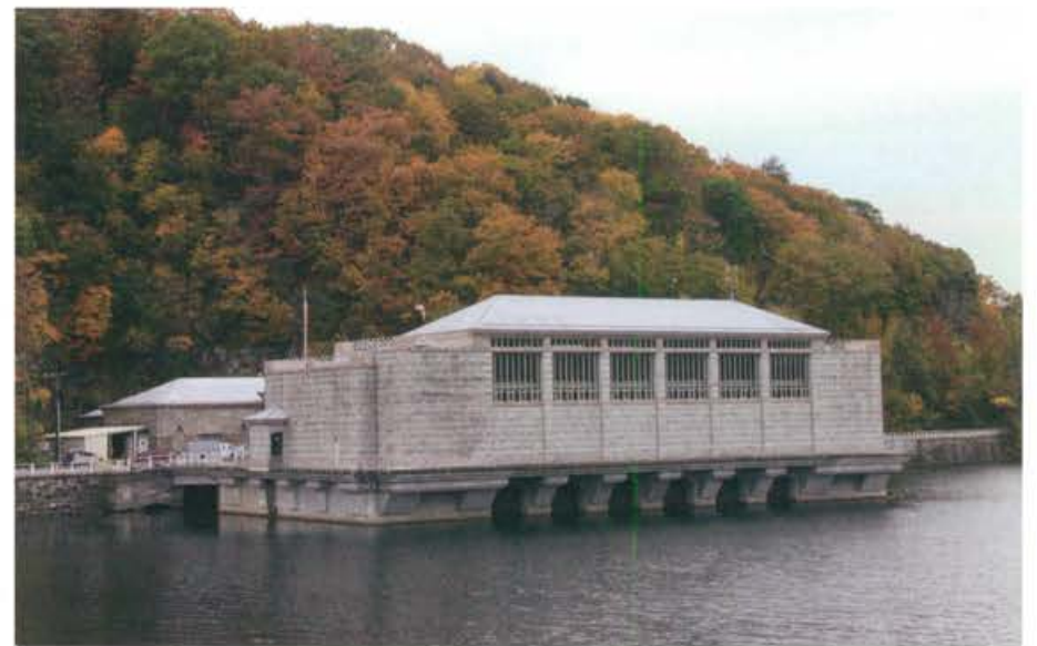
Ultraviolet Disinfection Facility
