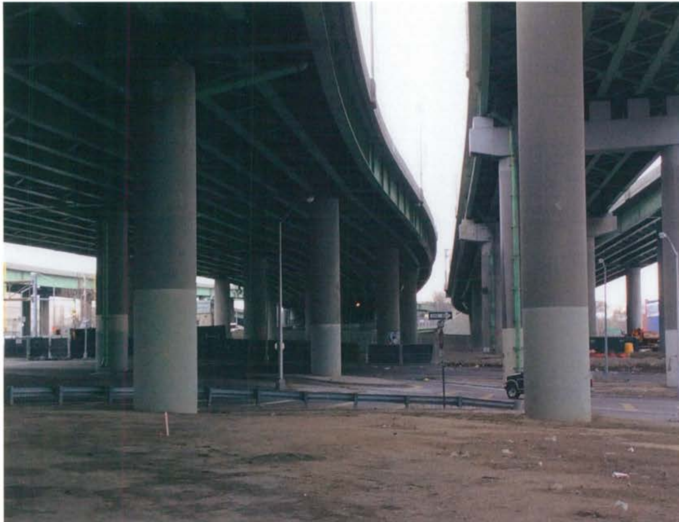
Cross Bronx crossing and Bruckner Expressways
