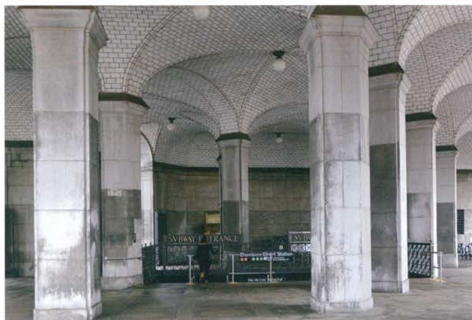
Manhattan Municipal Building Rotunda (Guastavino, 1915)
