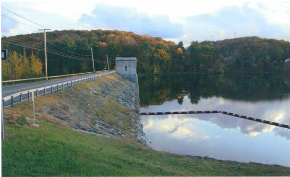
West Branch Dam (1891)
