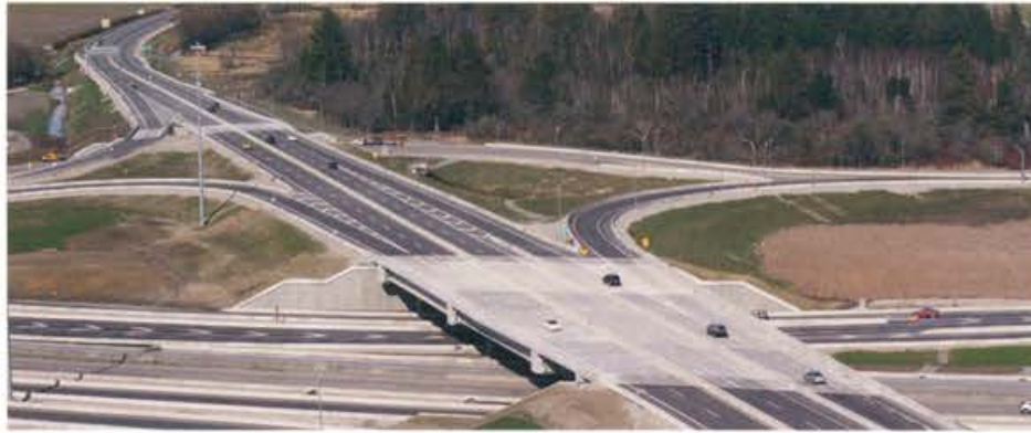
South Fraser Perimeter Road, Vancouver, Canada
