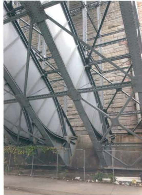
Washington Bridge (Schneider, 1889)
