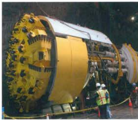
Second Avenue Subway
