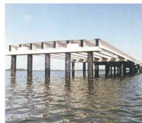
Teodoro Moscoso Bridge, Puerto Rico
