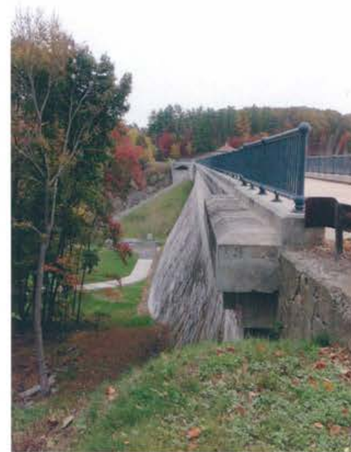
West Branch Dam (1891)
