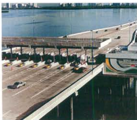
Teodoro Moscoso Bridge, Puerto Rico
