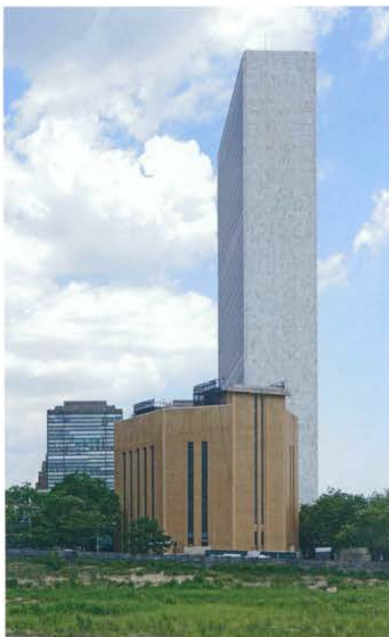
Midtown Tunnel, ventilation tower
