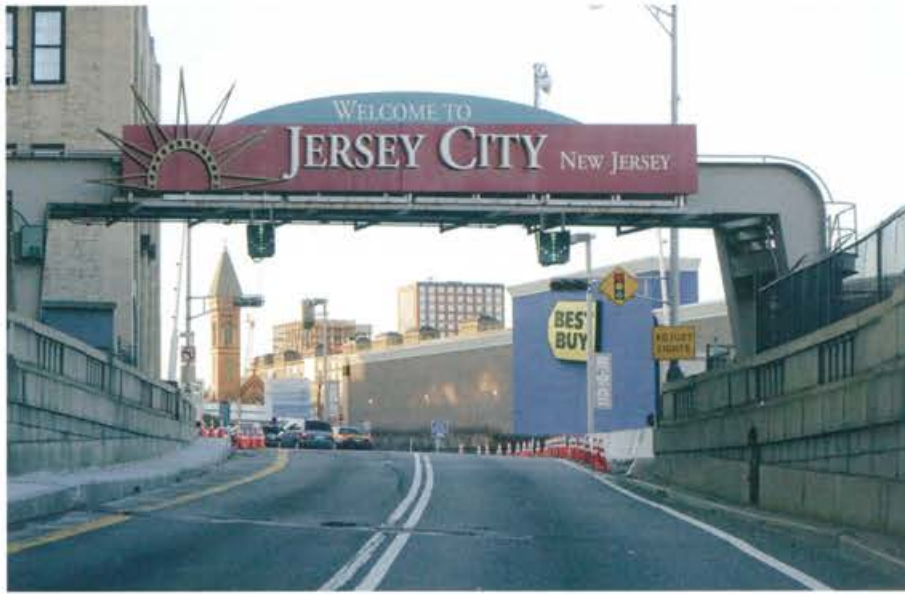
Holland Tunnel entrances
