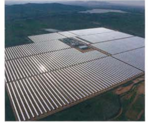
General area view Casablanca Solar Power Plant
