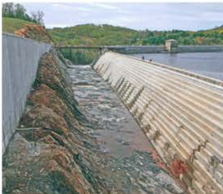
Croton Falls Dam, Westchester County, NY. 2012
