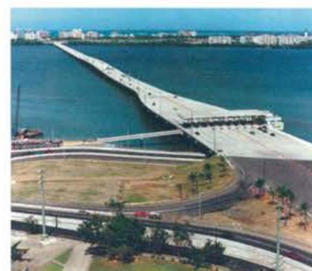
Teodoro Moscoso Bridge, Puerto Rico
