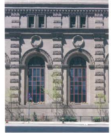
IRT Powerhouse (MM&W, 1904)
