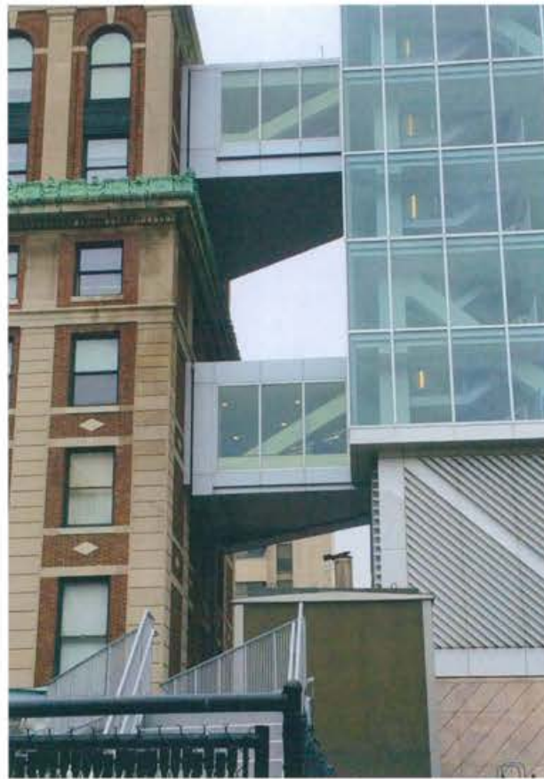
Northwest Corner Building (Moneo, 2010)
